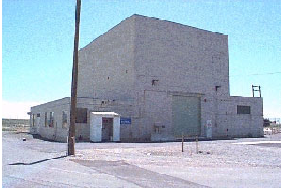
Figure 7. Mixed Waste Storage Facility
