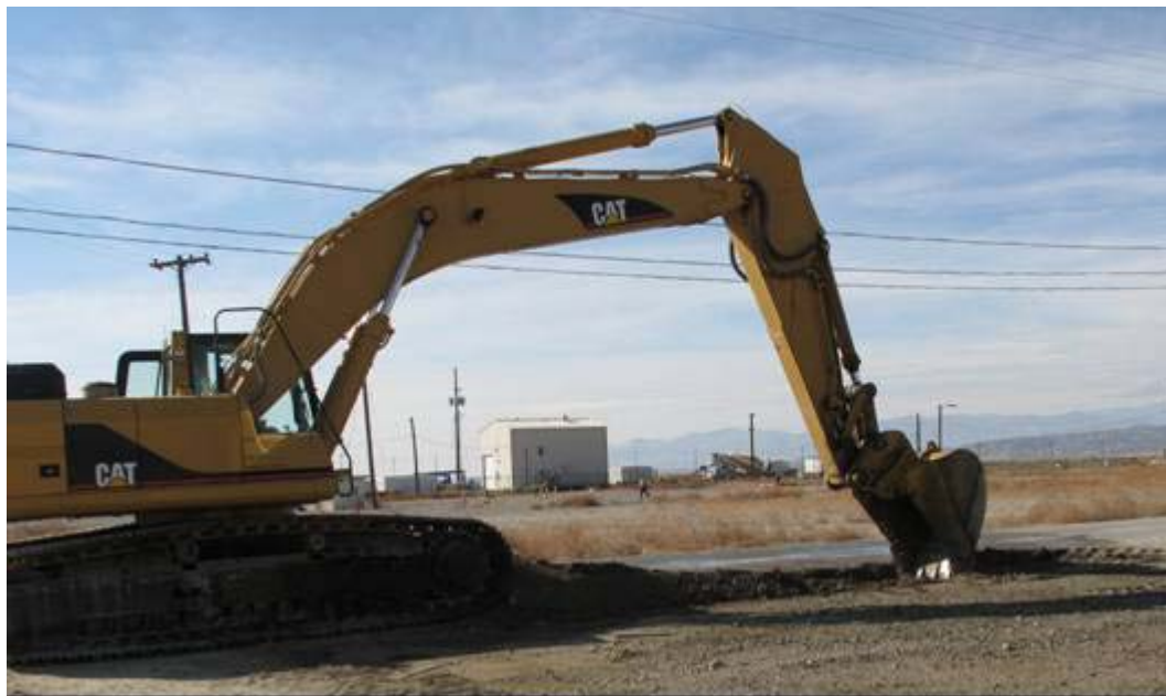
Fig. 5. Real-time remediation process showing the pre-excitation survey, marking of the excavation boundary, removal of contaminated soil.
