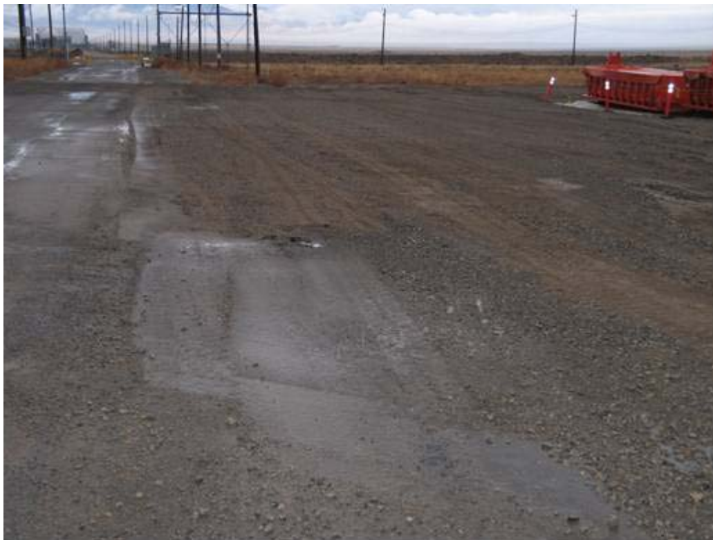
Fig. 5. Real-time remediation process showing post-excitation survey and the backfilled area.
