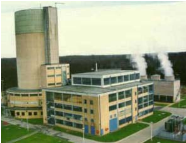
Figure 2-1: AVR – the first pebble-bed reactor.
