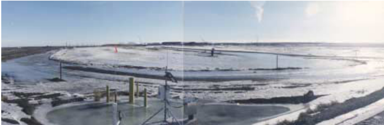
Figure D-2. Photograph showing ponding at the Subsurface Disposal Area resulting from an average snow melt over frozen ground.
