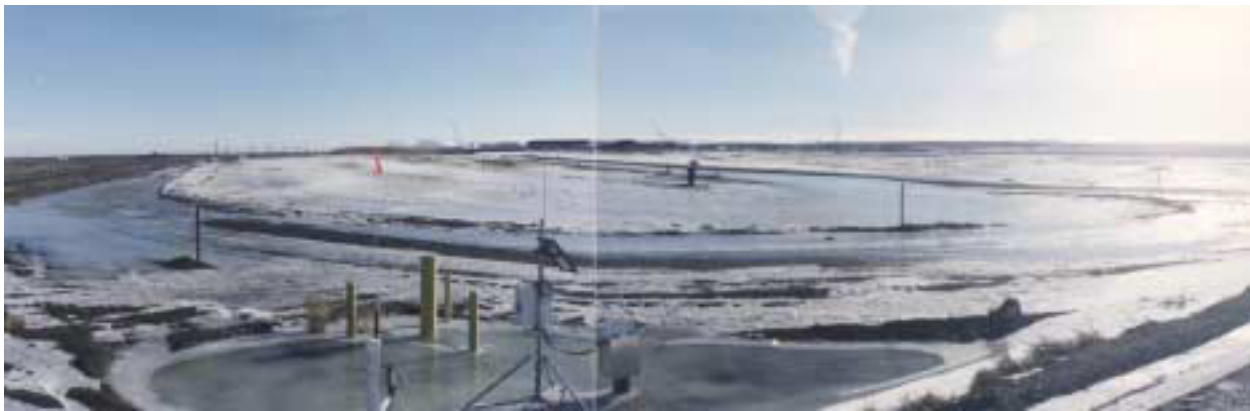
Figure 3-2. Photograph showing ponding resulting from an average snow melt over frozen ground at the Subsurface Disposal Area of the Radioactive Waste Management Area.
