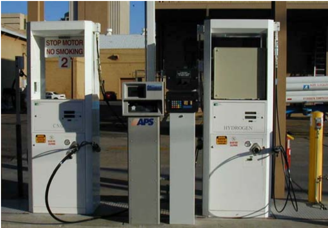
Figure 9. Compressed natural gas dispenser (left) and hydrogen and H/CNG fuels dispenser (right), with the two credit card interface pedestals in between.
