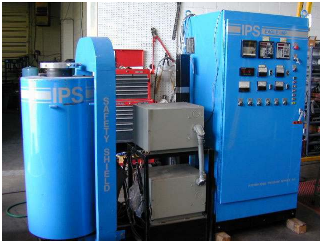
Figure 7. The Hot Isostatic Press being installed at the Idaho National Laboratory.
