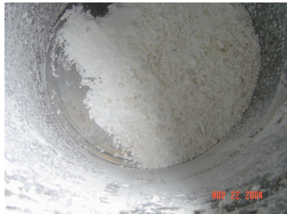
Figure 11. Visual inspection of ANL#1128.
