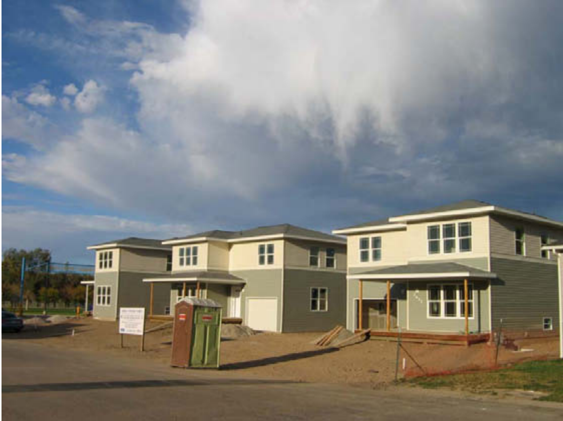
Figure 3. Building America prototype homes at Magna, Utah
