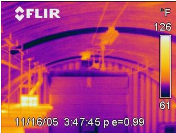
Figure 41 (IR0017) Warehouse Ceiling
