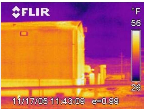
Figure 48 (IR0035) Southwest corner of the Gas Plant Office
