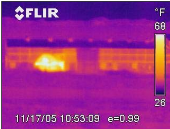
Figure 23 (IR0031) Northwest corner of Science Center.
