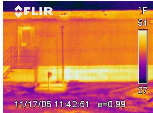
Figure 47 (IR0034) West door of the Gas Plant Office.
