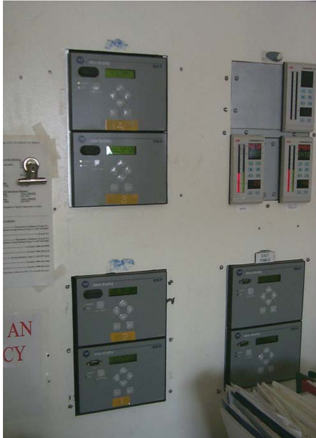
Figure 5 (PH0022) Allen Bradley Motor Protection (model 825-p)
