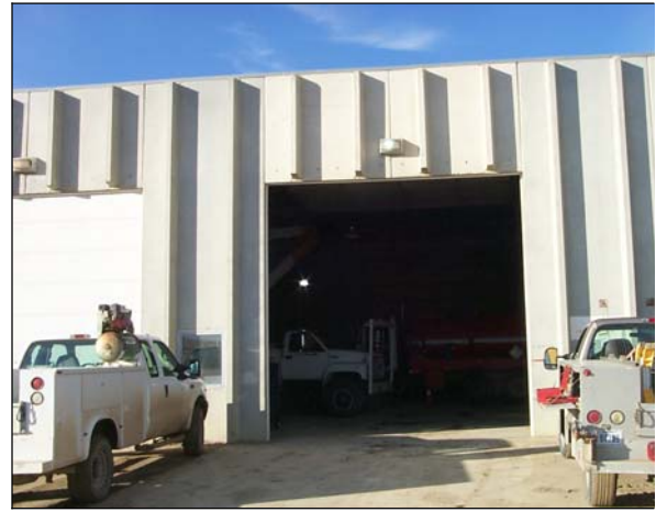
Figure 34 (PH0011) Front of the Shop area with 1 outside light on.
