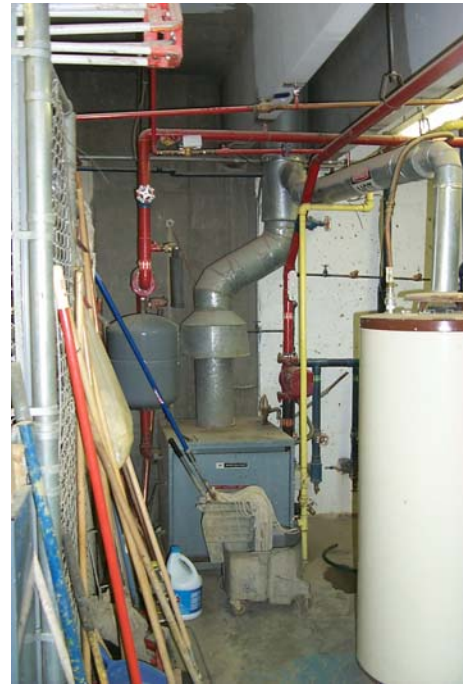
Figure 30 (PH0010) Un-insulated hot water lines.
