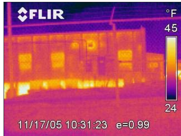
Figure 36 (IR0025) West Northwest corner
