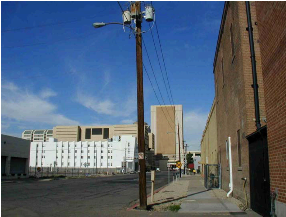
Figure 1.1. West Side of the APS Alternative Fuel Pilot Plant.
