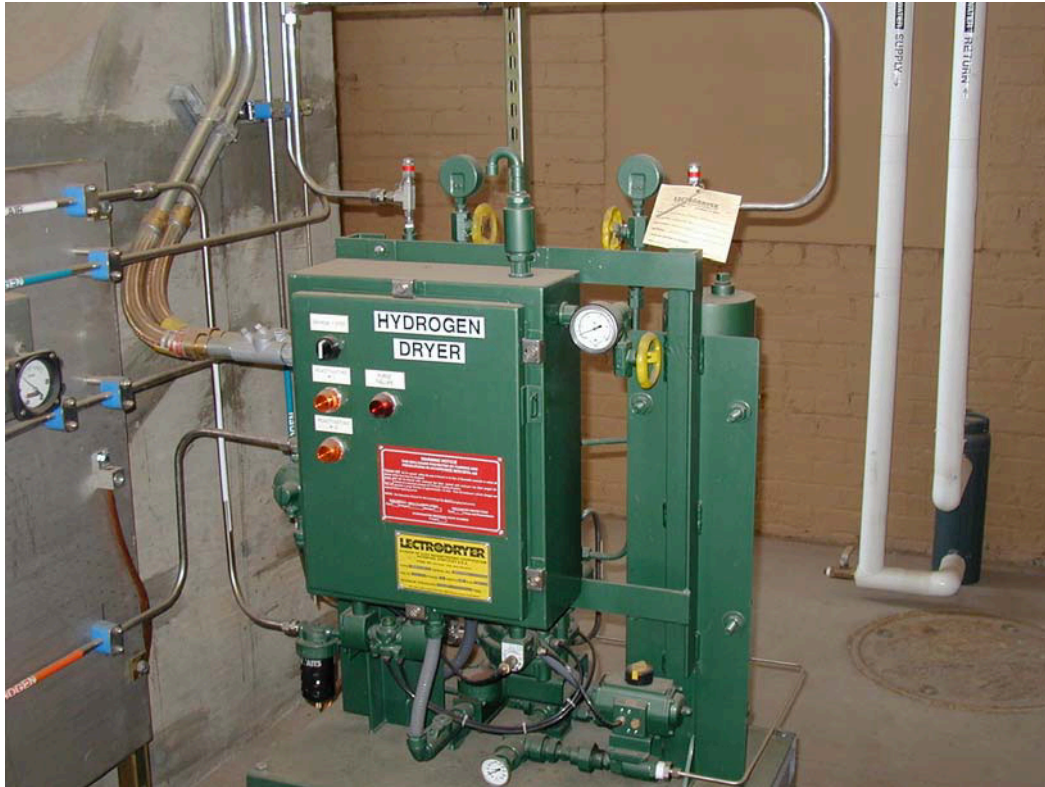
Figure 2.2. Lectrodryer hydrogen dryer.
