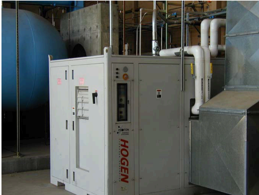
Figure 2-1. HOGEN 300 proton exchange system.
