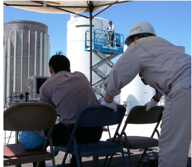
Fig. 11. CRIEPI and LAZOC Inc. representatives performed ultrasonic testing in August 2005.
