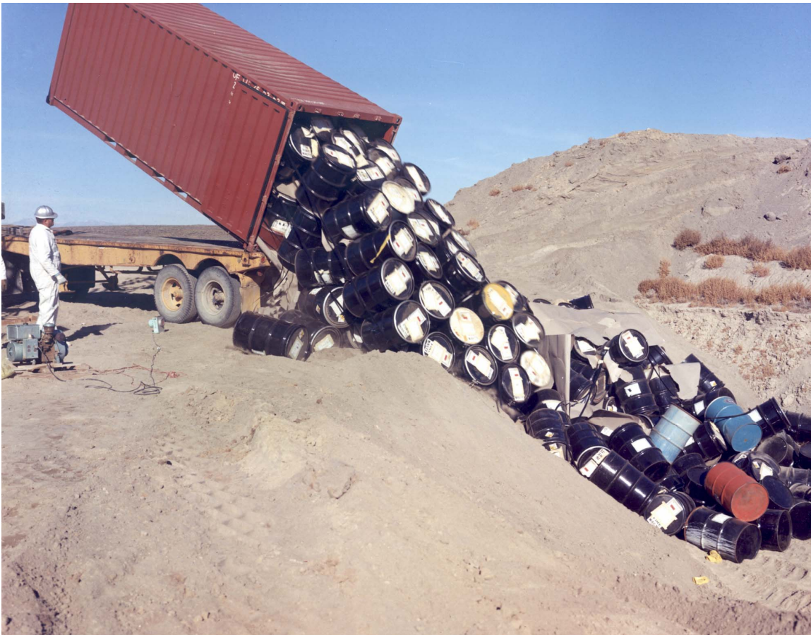
Figure 3-8. To reduce worker exposure times, random dumping practices were adopted in later years (INEEL photo # 69-6138).
