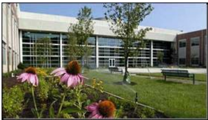
Courtyard for Events (Photo courtesy of ORNL)
