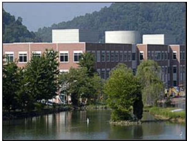
First LEED-certified facility in Tennessee (Photo courtesy of ORNL)
