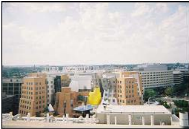
The Ray and Martha Stata Center (Photo courtesy of K. Kostelnik)
