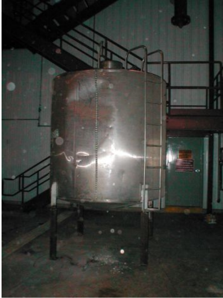
Figure 3.1.3 Vessel T-301 4,250 Liter HS/LE reactor (9'x 6' diameter-under construction)
