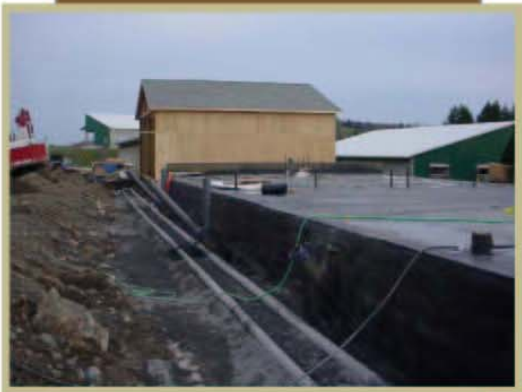
Digester and equipment building while under construction (11/21/05)
