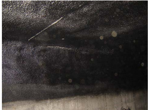
Figure 38. Inside view of the digester after the applications of polyurethane/polyurea to seal the gas chambers on both sides of the digester (picture taken on August 30, 2006).
