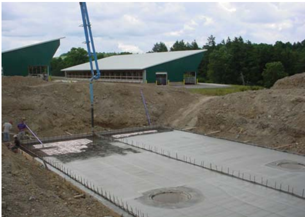
Figure 3. Concrete-pouring of the floor of the tank (picture taken on August 23, 2005).
