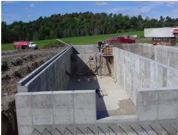
Figure 9. Close-up of one of the chambers of the effluent-side of the digester (picture taken on September 30, 2005).
