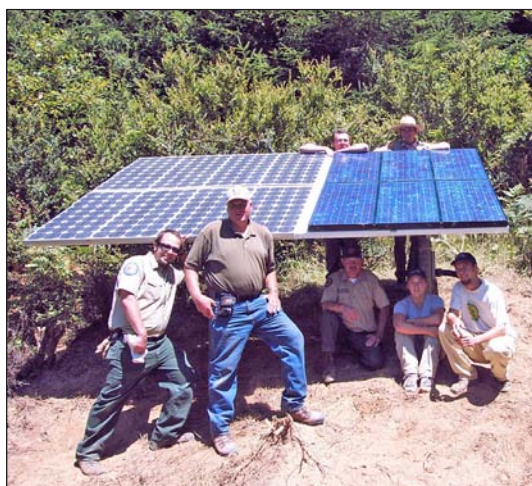
Interns Erin McDonald and Matthew Smith (lower right) pose with RNSP employees after successful installation of Espa Lagoon's new PV system.
