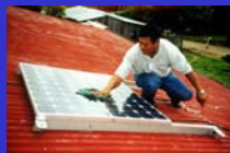
Ken Olson, DOE/NREL
