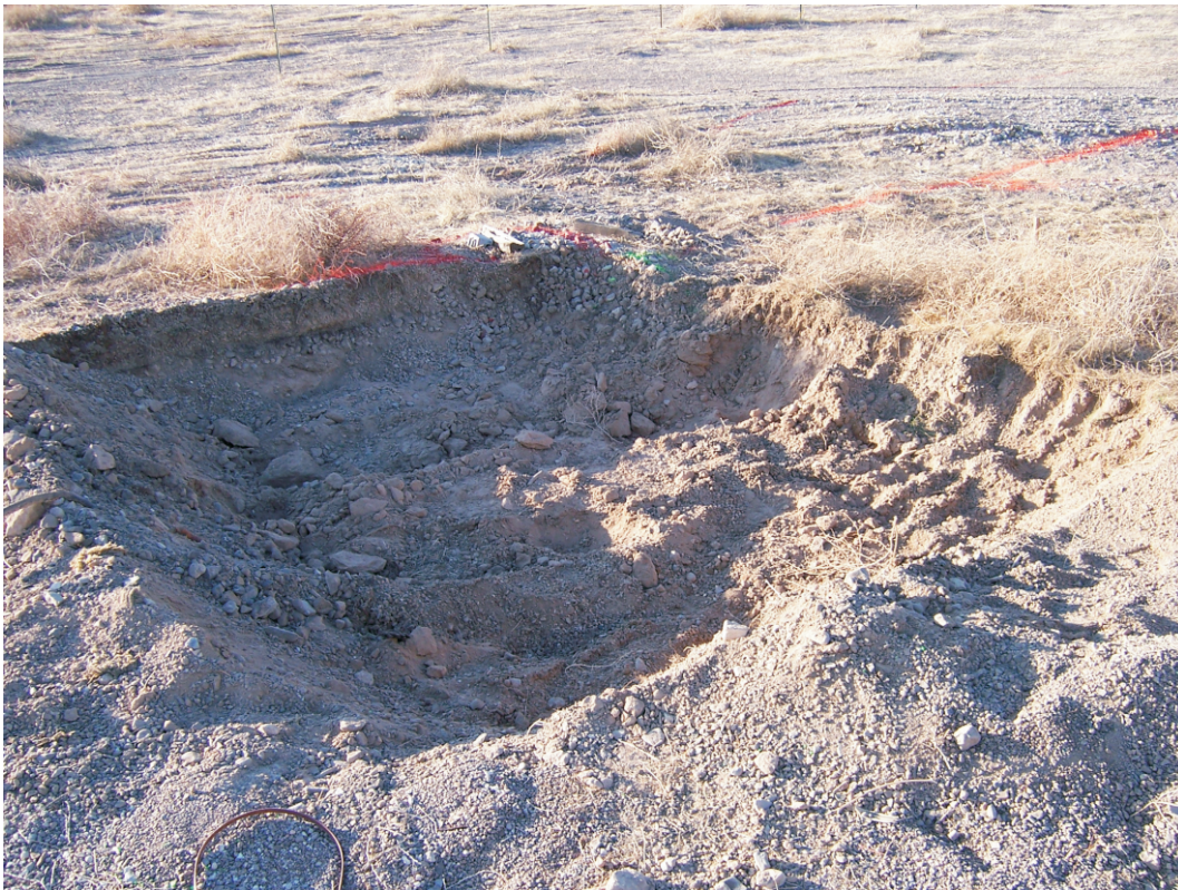
Photograph 2: Soil location during excavation (01/11/2007)
