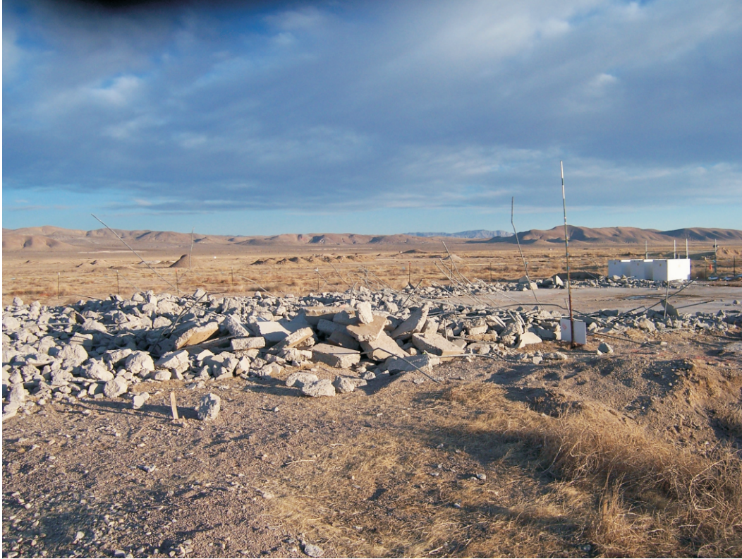
Photograph 5: Concrete pad location during corrective action (01/17/2007)
