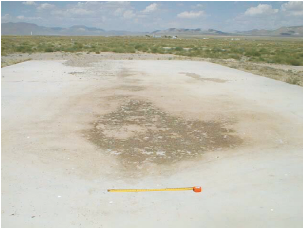
Photograph 1: Concrete pad location prior to corrective action (08/25/1998)
