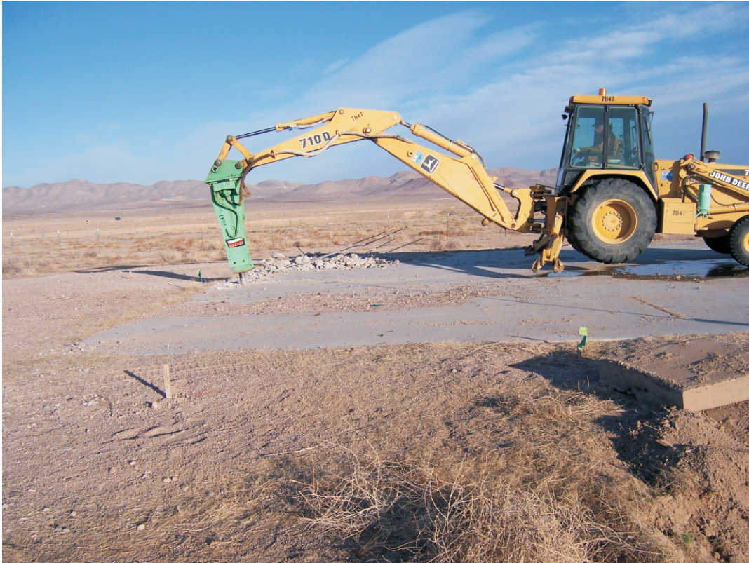
Photograph 3: Concrete pad location during pad breakup (01/11/2007)
