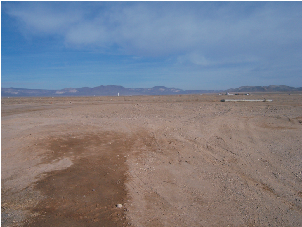
Photograph 6: Concrete pad location after corrective action (02/08/2007)
