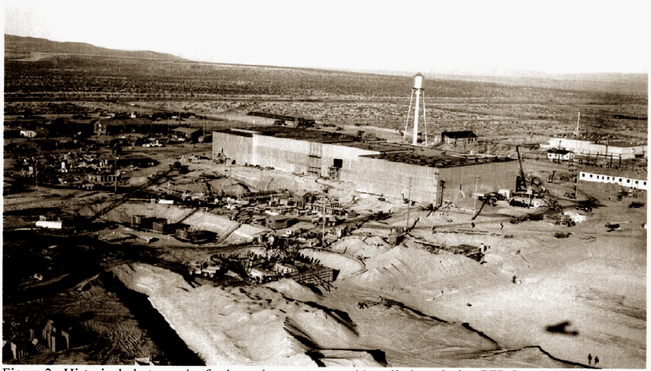
Figure 2. Historical photograph of sub-grade structures and installations during PFP Construction (Photo 1).
