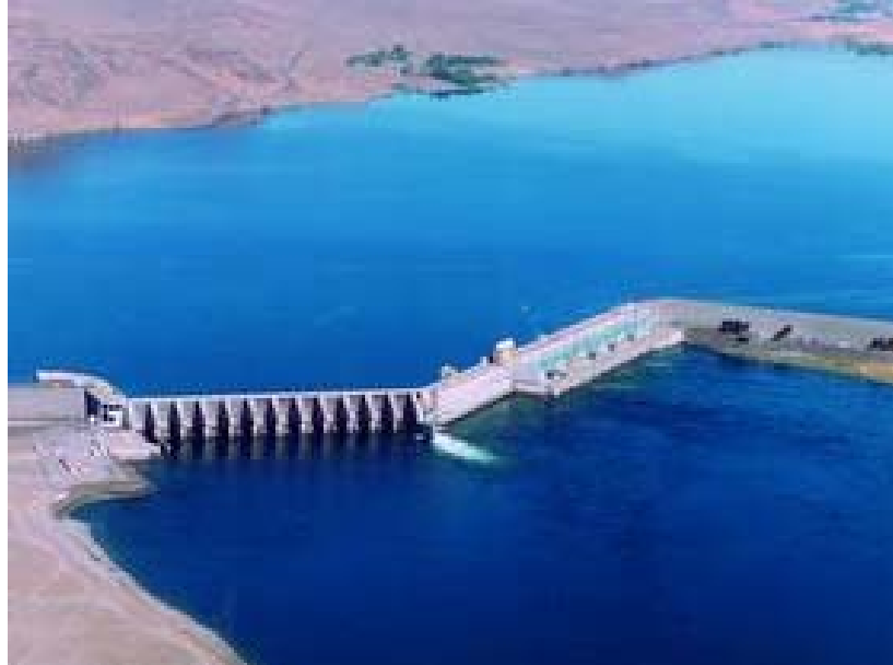
Figure 2.2. Wanapum Dam on the Columbia River, Washington. The spillway is on the left, the powerhouse is in the center, and the earth fill section is on the right.
