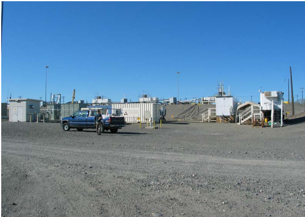
Figure B.12. Surface Conditions Around Borehole 299-E27-22 (April 19, 2007)
