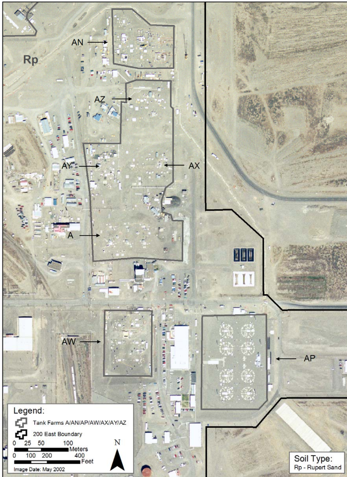
Figure 4.6. Waste Management Area A-AX. Also shown are double-shell tank farms AN, AP, AW, AY, and AZ. The tip of WMA C is just visible in the upper left corner of the image.
