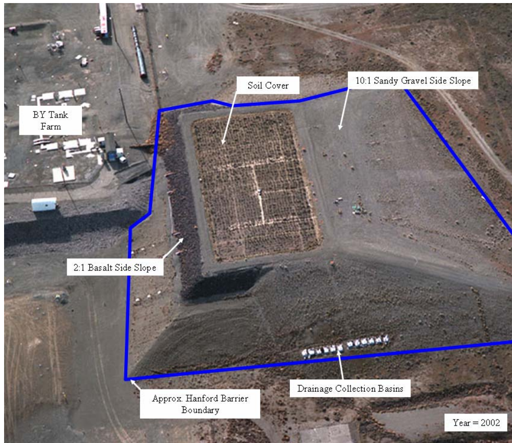
Figure A.5. Aerial View of the Prototype Hanford Barrier Looking in Southerly Direction. Image captured in 2002.
