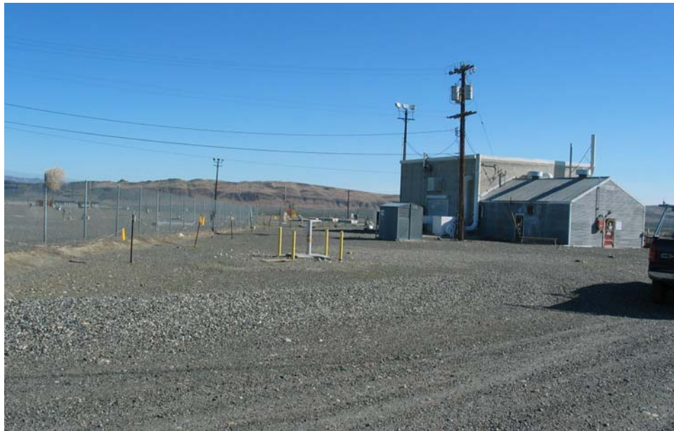
Figure B.8. Surface Conditions Around Borehole 299-E33-338 (April 19, 2007)
