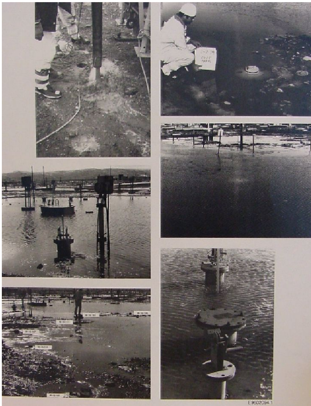
Figure 4.4. Temporary Flooding Above T Farm Following Rapid Snowmelt Above Frozen Ground (after Hodges 1998). Photograph is dated February 7, 1979. Hanford Meteorological Station weather records show air temperatures in January 1979 averaged -10.6^{\circ}\text{C} ( 13^{\circ}\text{F} ), and on only one day did the maximum air temperature exceed 0^{\circ}\text{C} ( 32^{\circ}\text{F} ).
