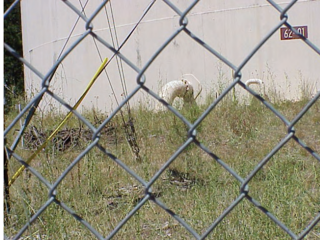
Figure 3. External rigid piping connection (nozzle).
