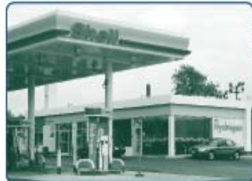
The Shell hydrogen fueling facility in Washington, D.C., is now one of a handful of such stations in the United States, and it most will likely be built in the near future. Local jurisdictions can benefit greatly from the experience of other local authorities who have already gone through the permitting process.
