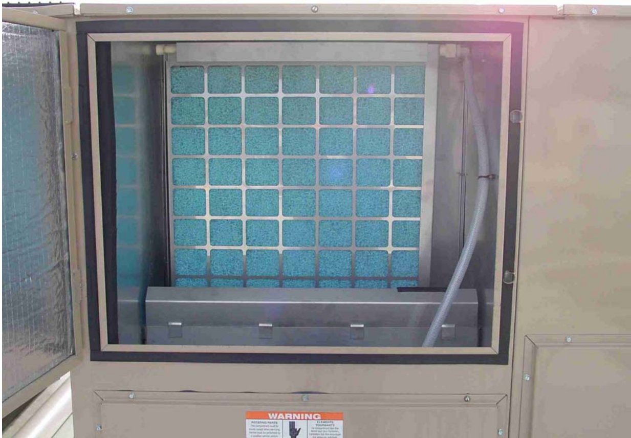
Figure 6. GEG Inventor 1400 Series Evaporative Media
