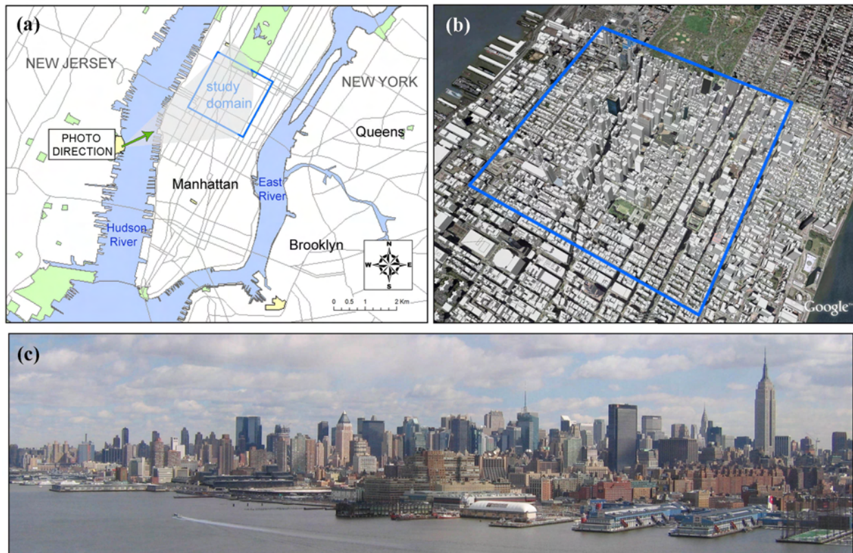
Figure 3.1. MID05 Study Area in Manhattan. The blue box in Panel (a) shows the 2-km-by-2-km MID05 study domain, and Panel (b) shows the domain in an aerial perspective of Midtown Manhattan extending from the Hudson River on the west to the East River on the east. The domain is just south of Central Park. The skyline of the Midtown study area is shown in Panel (c) where the photograph is taken from the Stevens Institute of Technology in New Jersey. Panel (a) shows the photograph direction.
