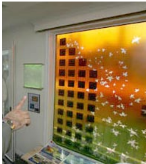
This house from the Solar Decathlon incorporated thin film PV in its windows. Photo courtesy of Wendy Butler-Burt of the U.S. Department of Energy.
