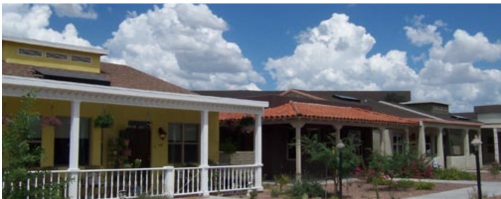
Copperheart Integrated Collector Storage water heaters are included on each JWM house. Photo courtesy of the Solar Store.
