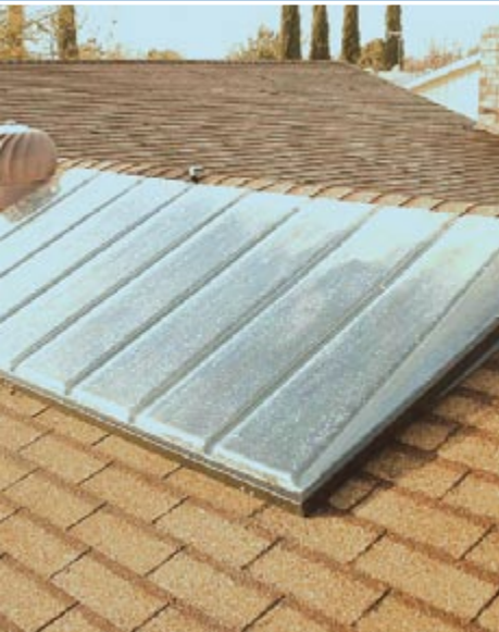
(left) Recent Innovations: Davis Energy Group is working with SunEarth and NREL to develop polymer-based ICS. Photo courtesy of Jay Burch of NREL.
