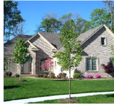
Home with PV shingle system. Photo courtesy of Decker Homes.
