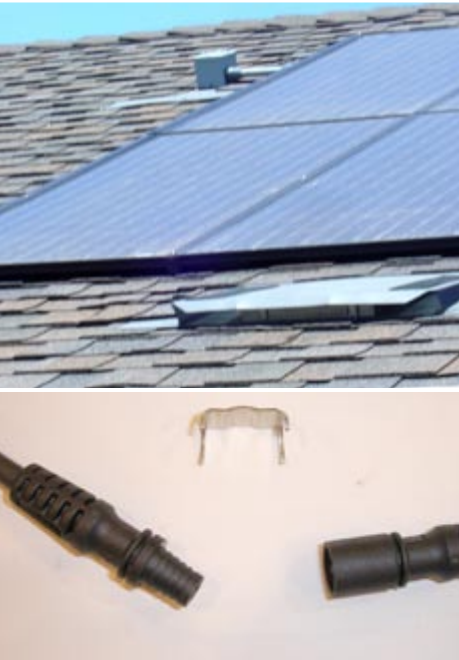
Photos of finished (top left) and roughed-in exterior junction boxes (right) offer an example of how roof flashing attaches to these PV system components.
