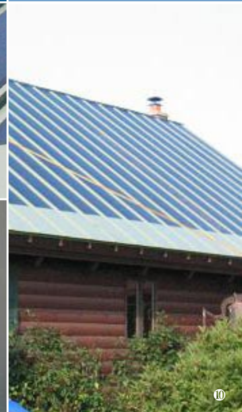
(photo series) Metal standing seam roof laminate systems step-by-step installation. Photo courtesy of Decker Homes.
