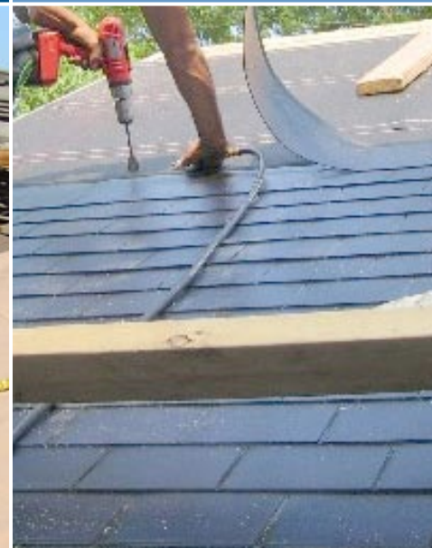
Building Integrated PVs are products that produce electricity from solar power while serving as a construction material, such as roofing. (right) Photo courtesy of Decker Homes.
