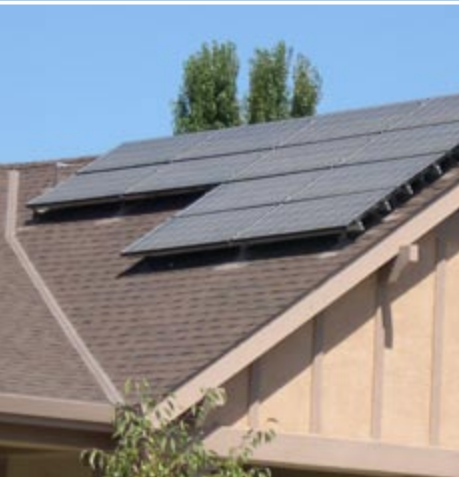
Clarum is building four zero energy research homes at Borrego Springs, California. Photos courtesy of Clarum Homes.
