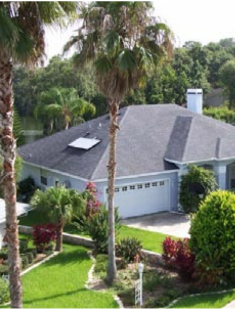
Solar thermal collectors in Florida and California.
