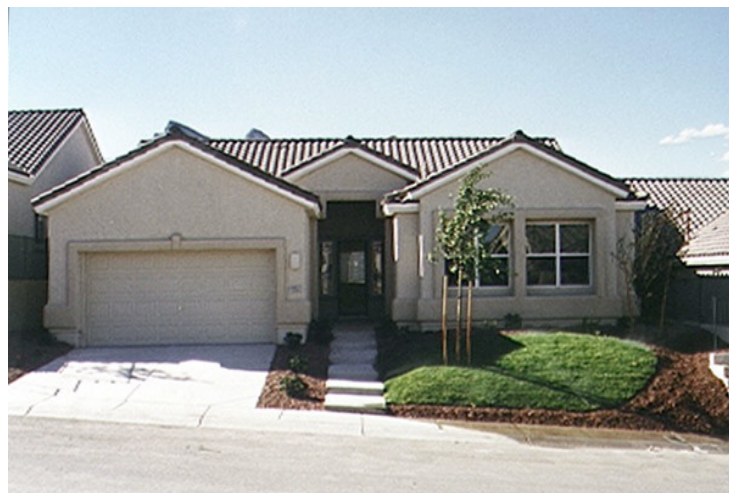
Figure 3. Home used for isothermal CFD case study (Cases 1-7), built by Pulte Homes in Las Vegas, Nevada. Courtesy of the Building America Program [17].
