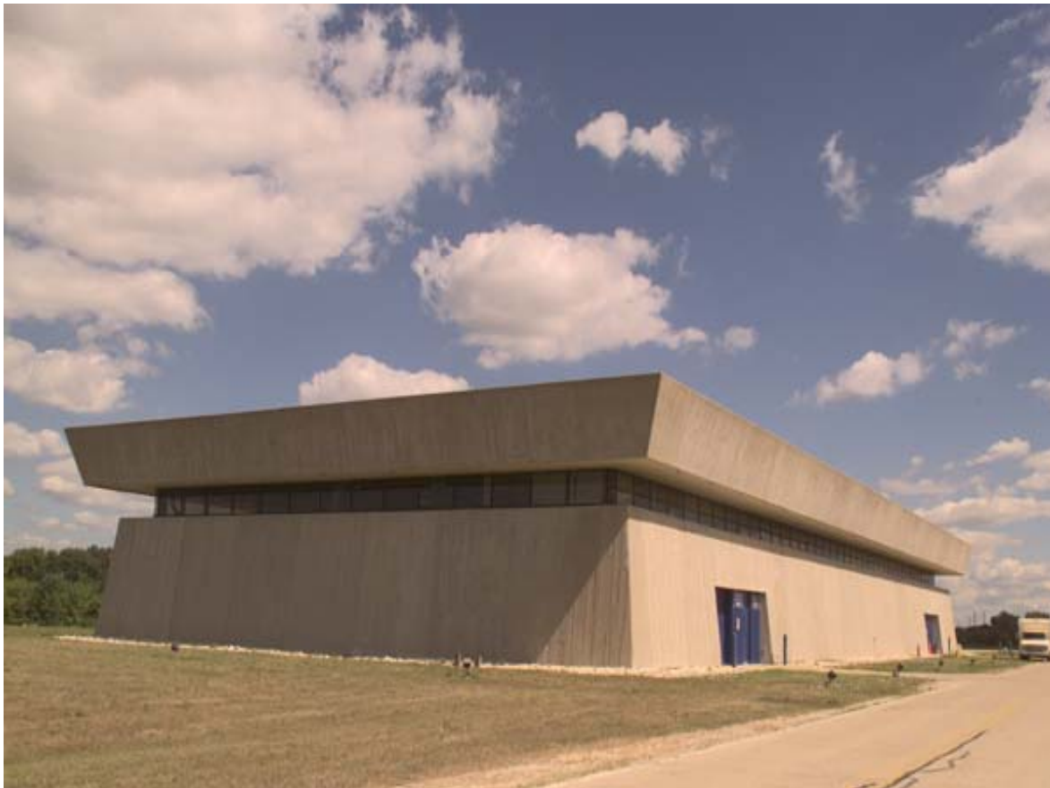
FIGURE 4. New Muon Lab Building.
