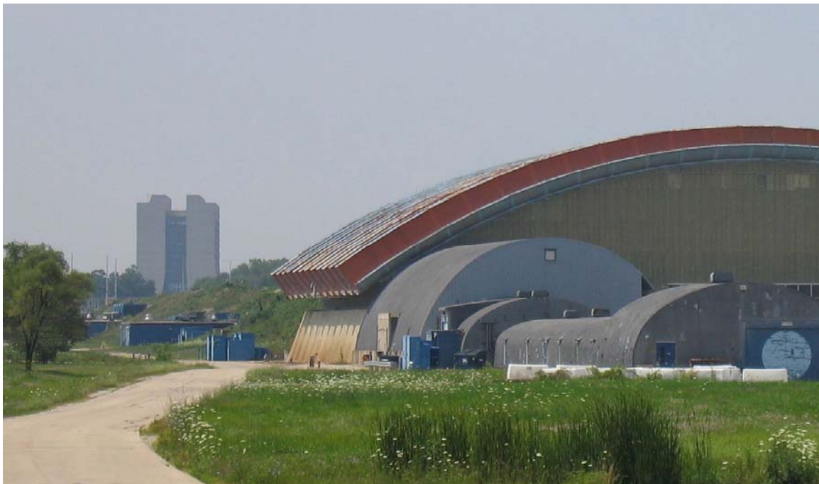
FIGURE 2. Meson Detector Building.
