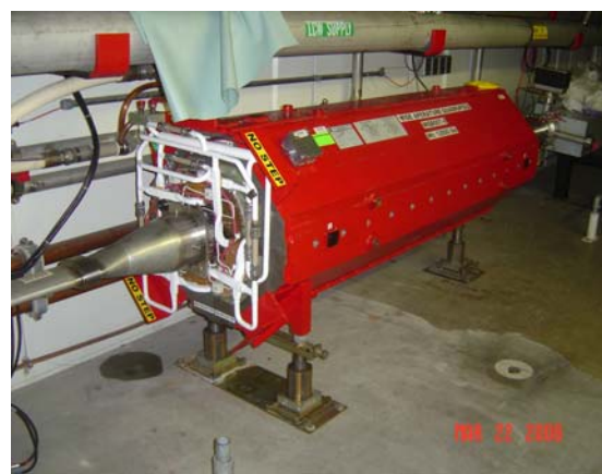
Figure 3: A WQB installed at the Q222 location.
