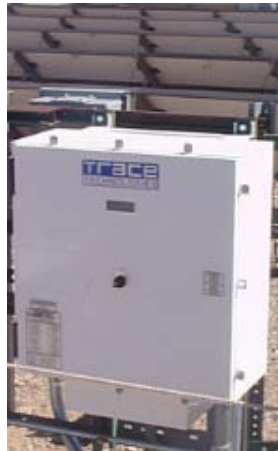
Figure 1. Xantrex PV20208 Grid-Tied PV Inverter
