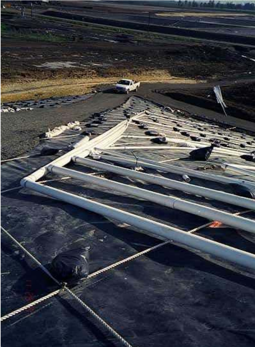
Image 23. Each LFG collection well has a dedicated collection lateral.
