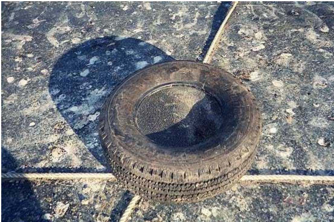
Image 49. Sandbag is covered by a tire and piece of geomembrane
