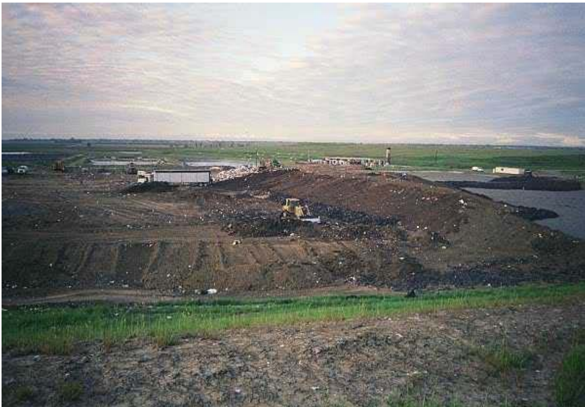
Image 4. Waste placement in lift 2 on the northeast 3.5-acre cell, April 2001
