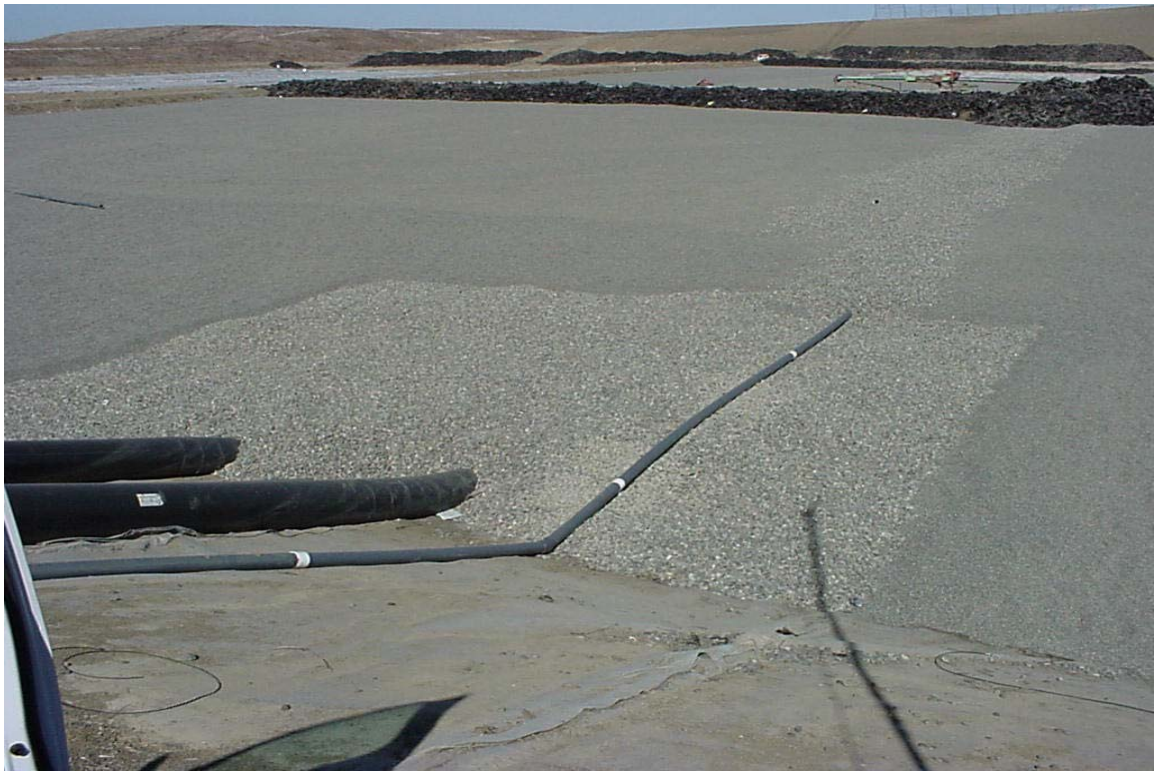
Image 16. Gravel drainage layer and leachate collection sump.
