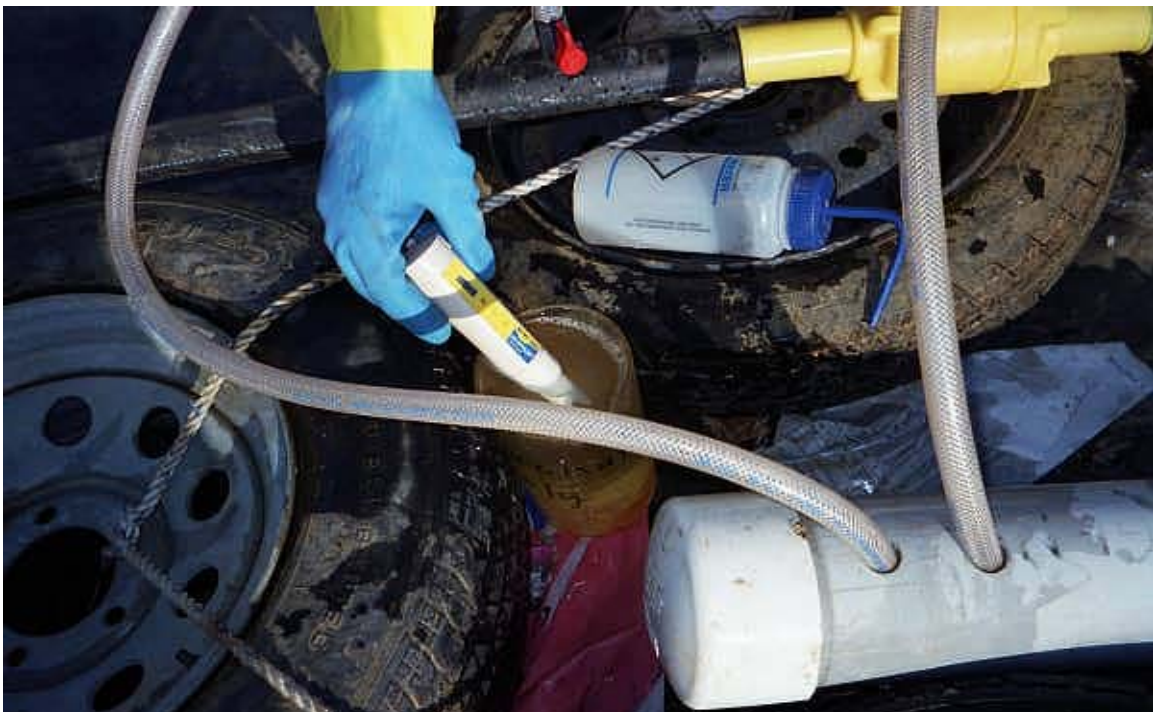
Image 42. The citric acid solution was monitored for pH as it passed through the injection laterals. As the citric acid displaced the groundwater in the injection lines, the pH dropped to approximately 4 and the injection lines were closed. The injection lines were flushed with groundwater the following day.
