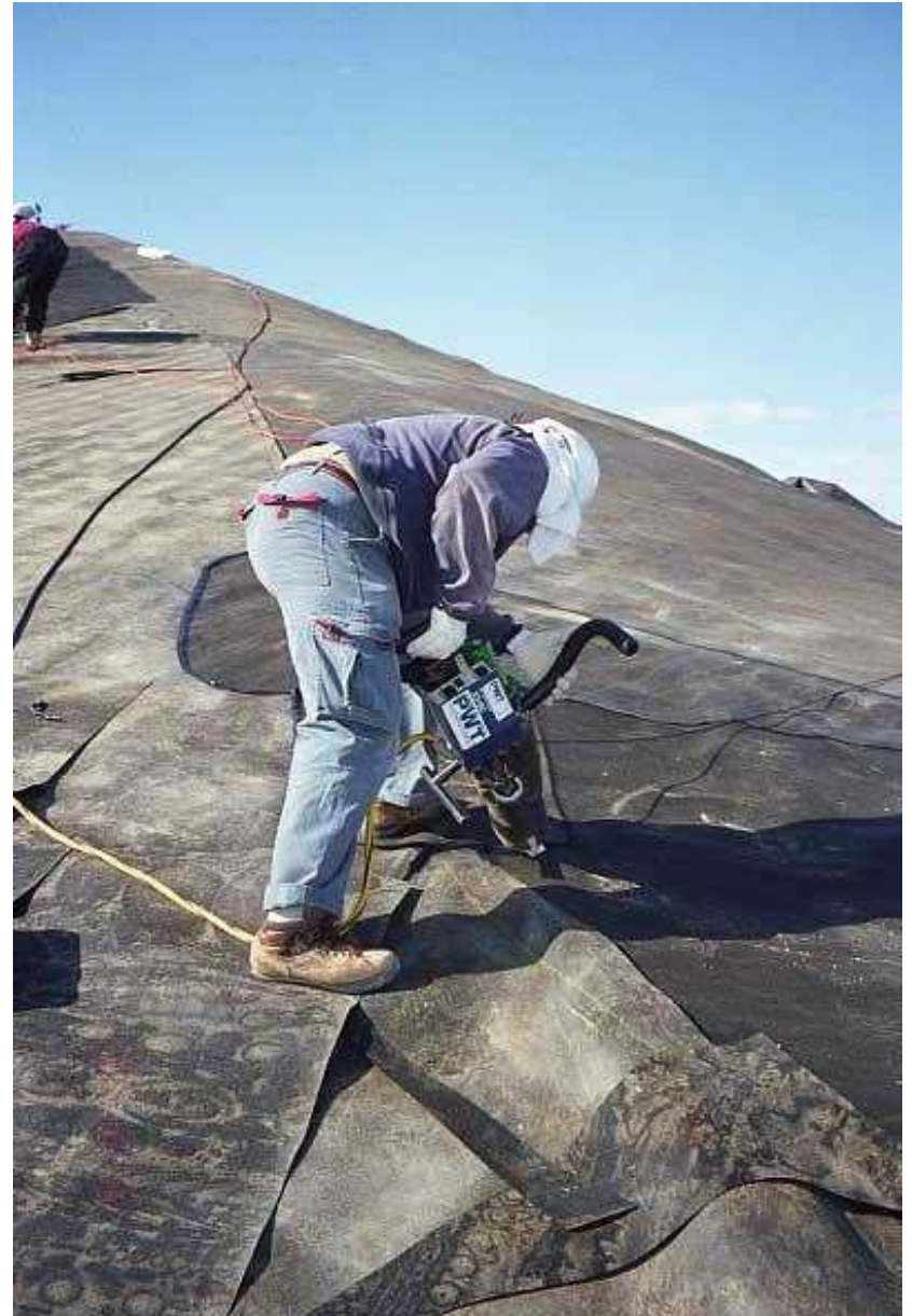
Image 30. Detail work around boots, corners, or patches required extrusion welding.
