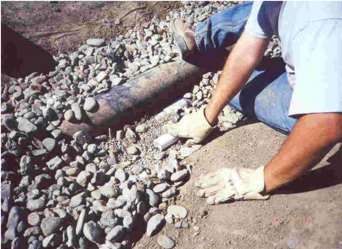
Image 2. Pressure tubes installed in LCRS trench
