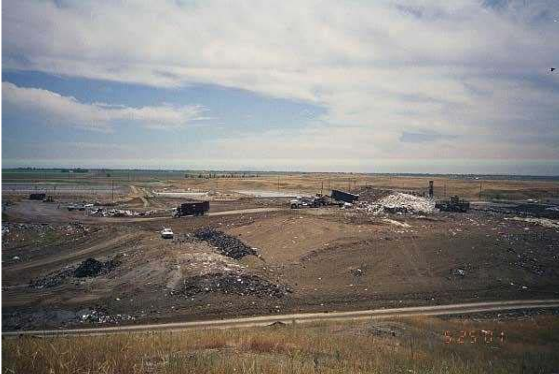
Image 5. Waste placement in lift 2 and 3 on the northeast 3.5-acre cell, May 2001
