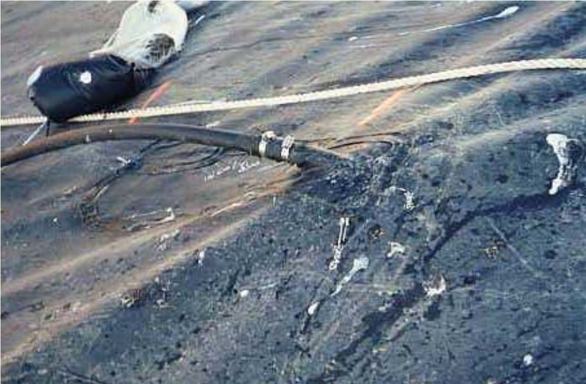
Image 19. Each liquid addition pipe was sealed to prevent air intrusion.
