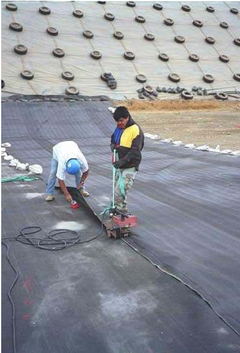
Image 29. The edges of each of the geomembrane panels were double-wedge welded.
