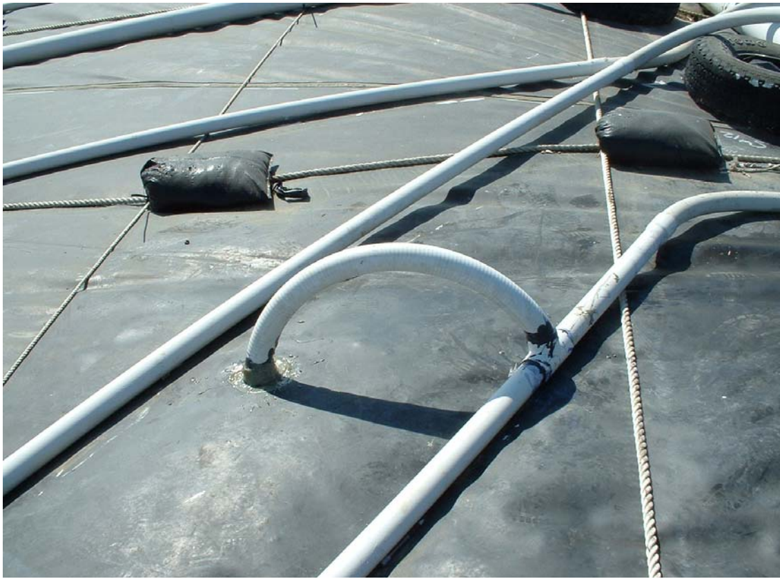
Image 45. Perforated piping installed below the surface liner on the northeast 3.5-acre cell to increase gas collection.
