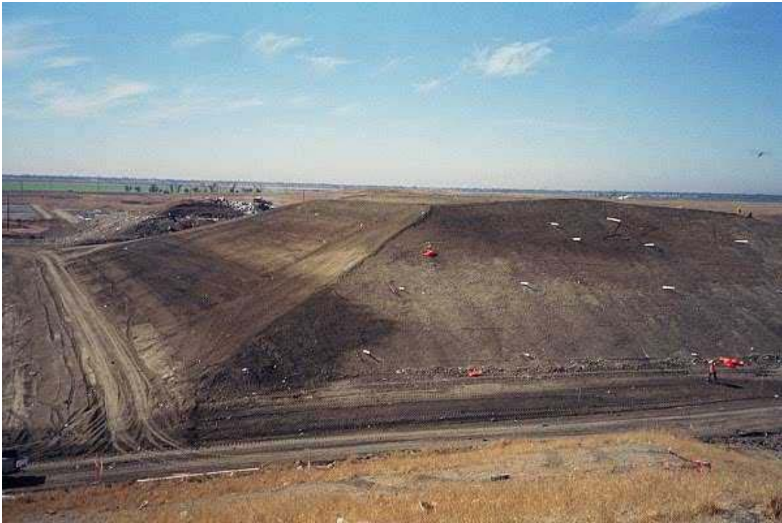
Image 7. Northeast 3.5-acre cell ready for surface liner installation, September 2001
