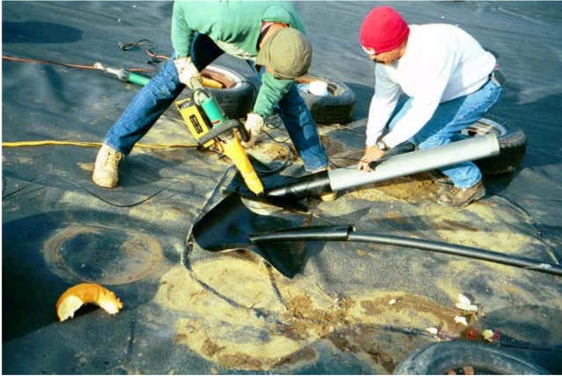
Image 51. Permanent geomembrane boot installation.
