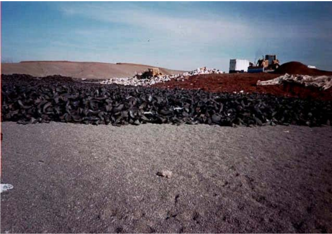
Image 1. Operations layer of the base liner consisting of shredded tires.
