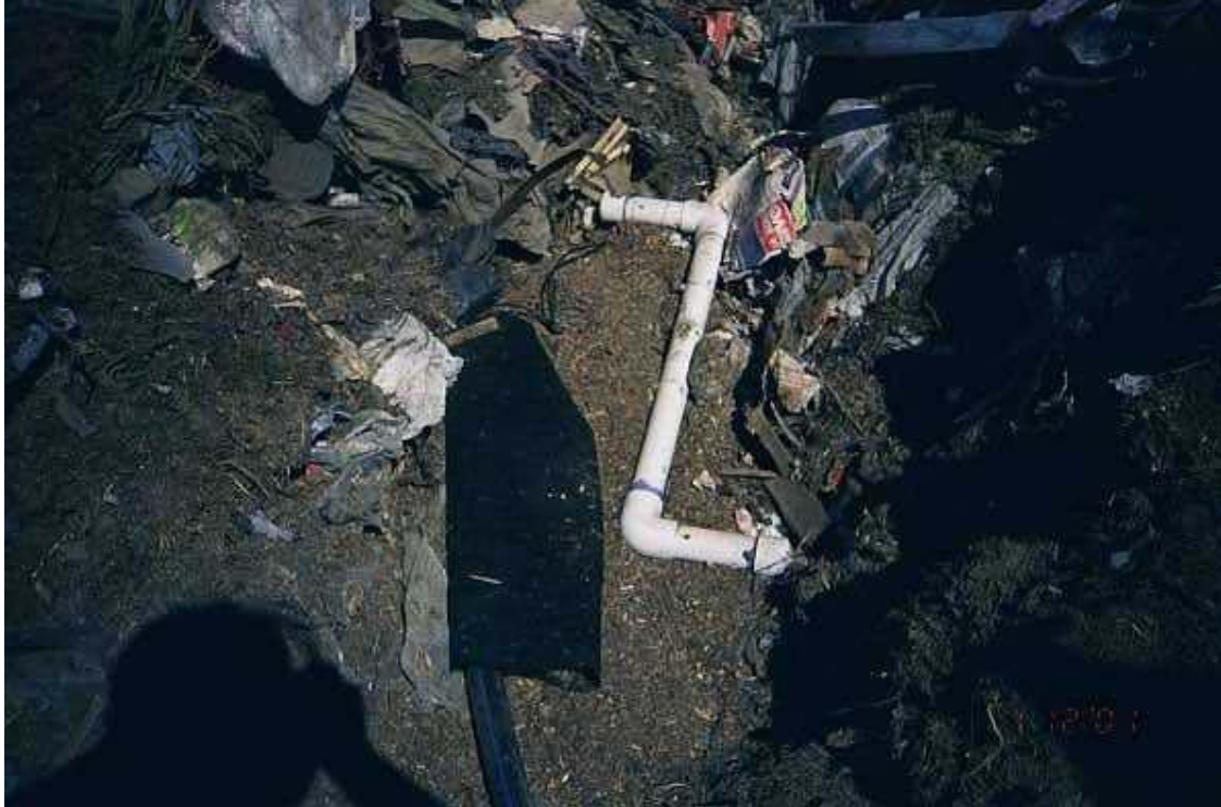
Image 2. Moisture, temperature, and tube installation
