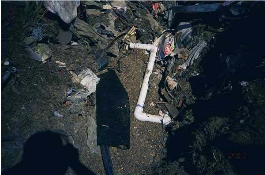
Image 15. Moisture, temperature, and tube installation
