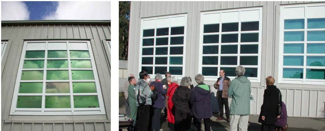
Figure 3. Exterior views of prototype EC windows at the fully tinted state (left and right photos) and a conventional spectrally-selective Azurlite window with interior Venetian blinds on the far right.
