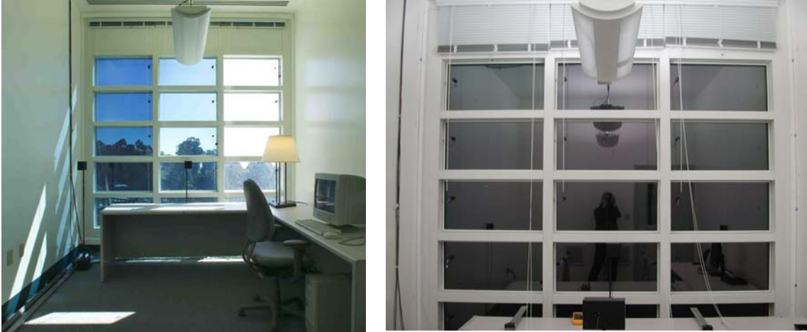
Figure 4. Interior views of the EC window wall with a) EC window at darkest, intermediate, and clearest states during the day (left) and b) EC window at its darkest state at night (right). The LBNL-installed sensors on the glass are not part of the EC product.
