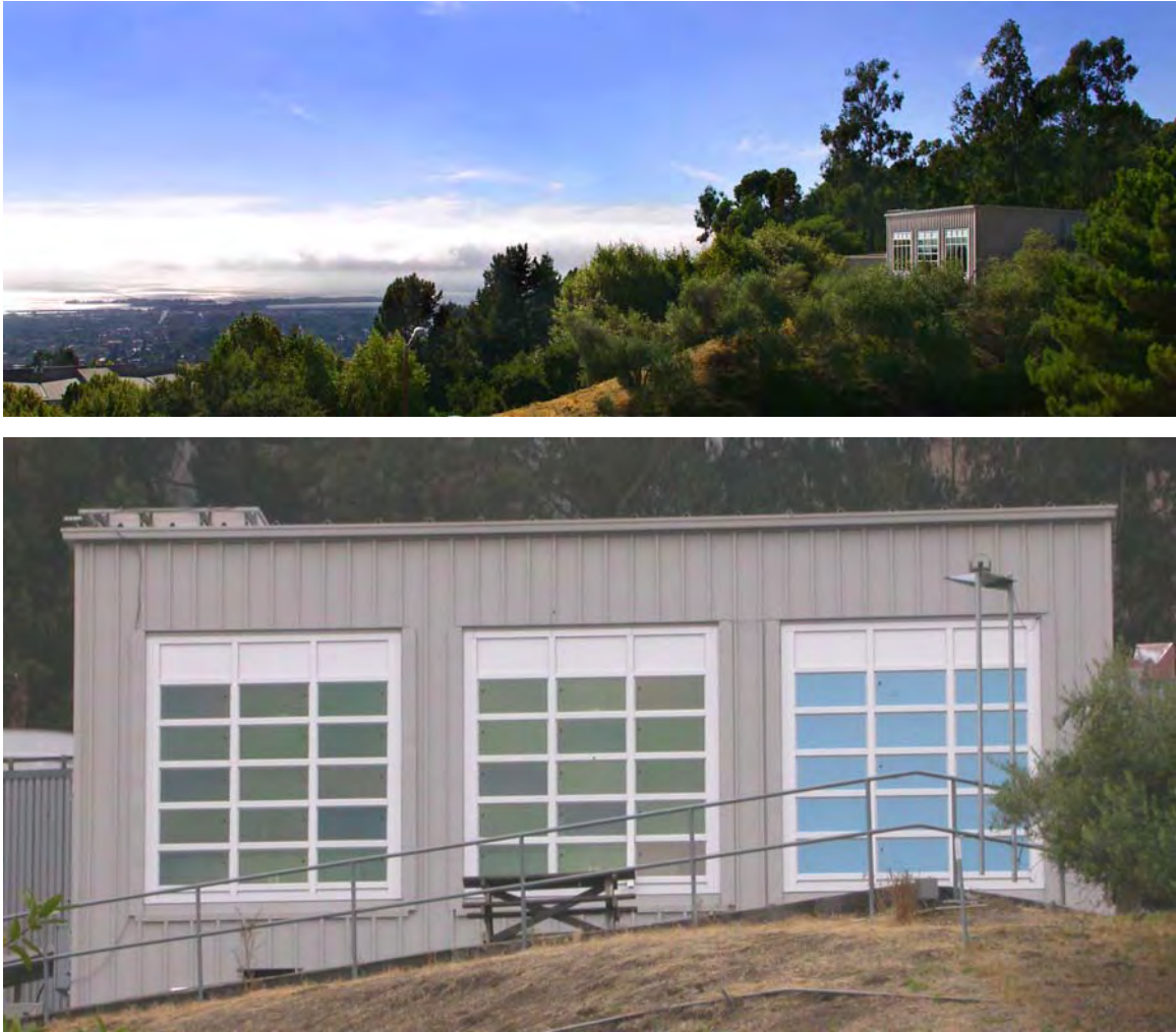
Figure 2. LBNL Window Testbed Facility (upper photo). South elevation of EC facades (middle and left) and spectrally selective low-e façade (right) on August 20, 2004 (lower photo).
