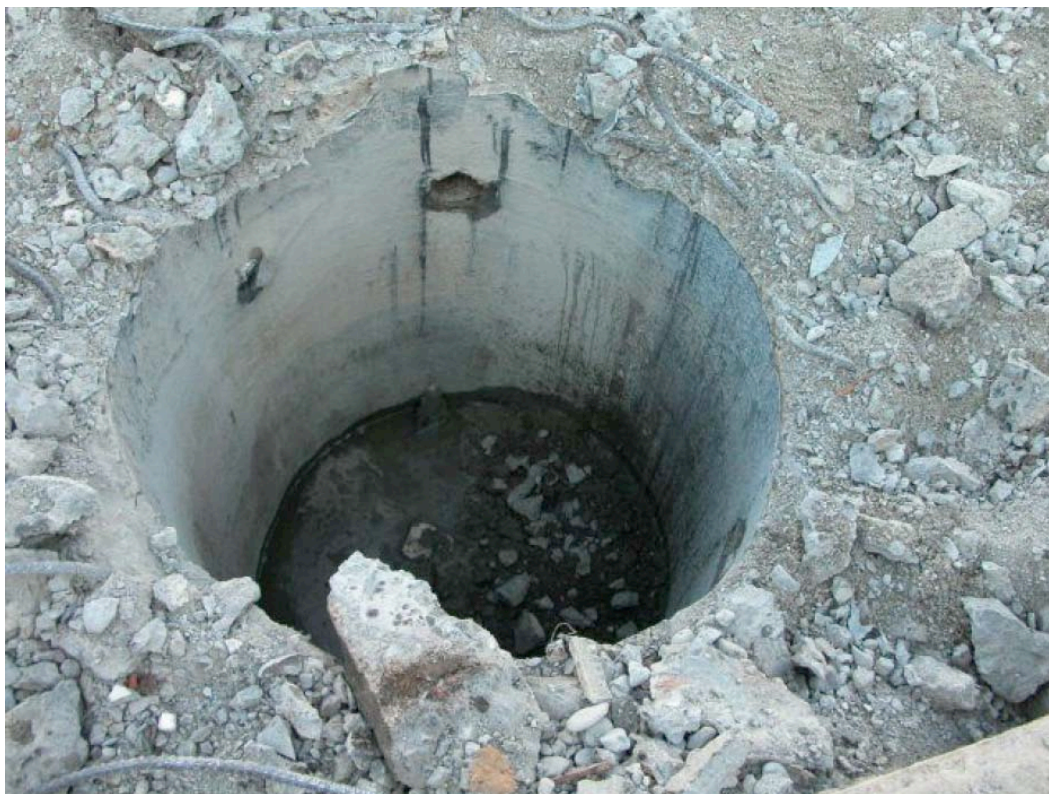
Figure 4-4. The In-Ground Sump Found in the Building 514 Filtration Room
