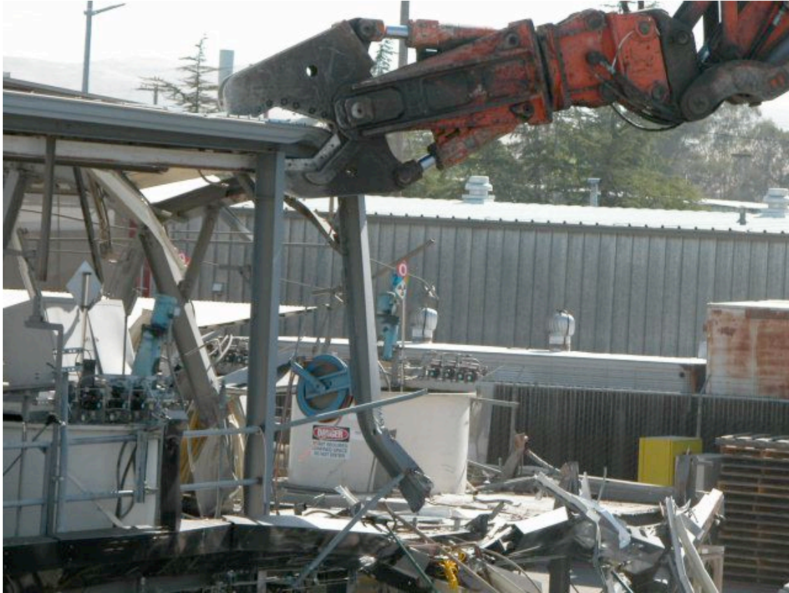
Figure 4-6. Wastewater Treatment Tank Farm Demolition
