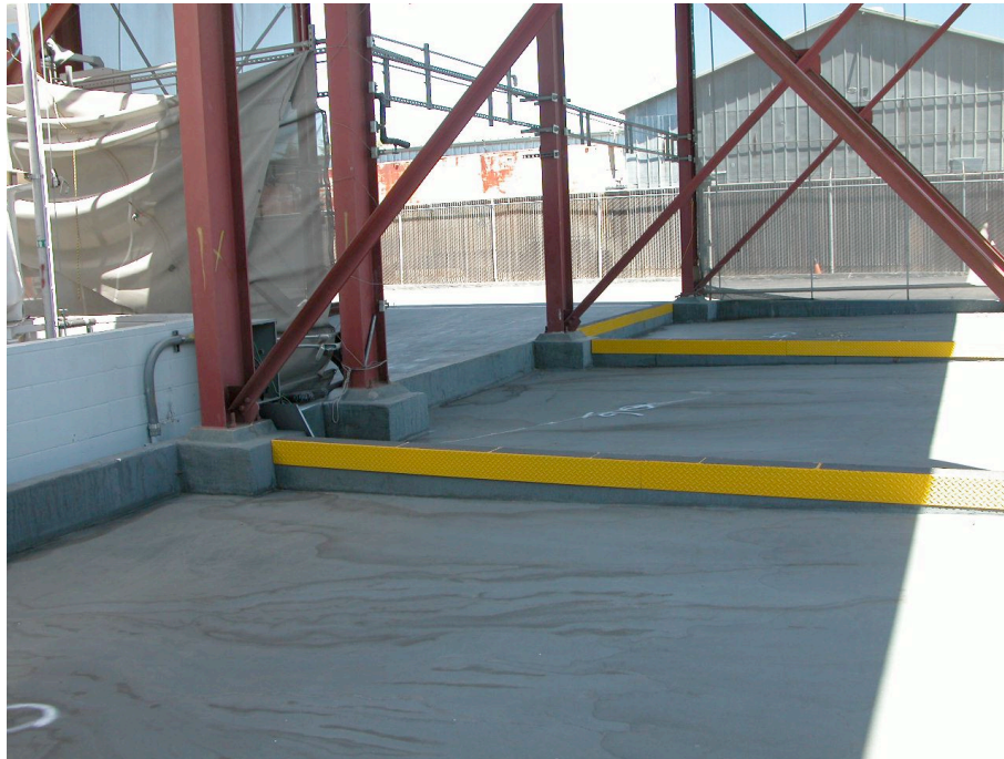
Figure 3-9. Area 514-2 Container Storage Unit
