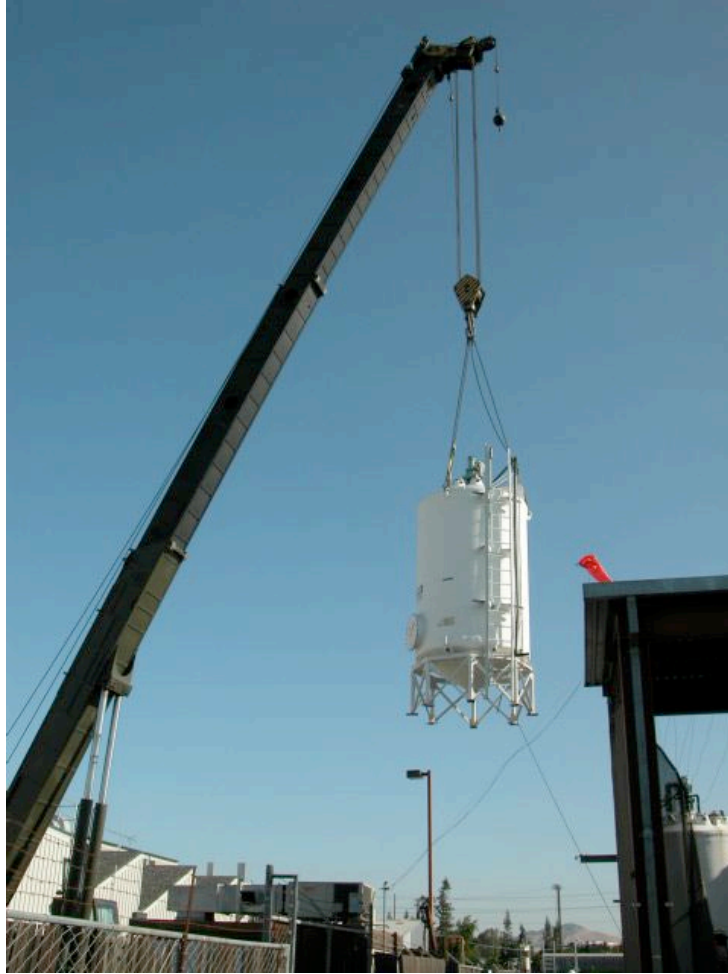
Figure 4-7. Quadruple Tank Unit Removal
