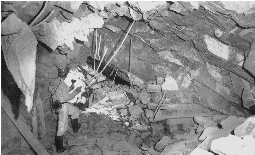
Ground failure in a South African gold mine under a rock burst (Courtesy of D. Ortlepp, 2003)
