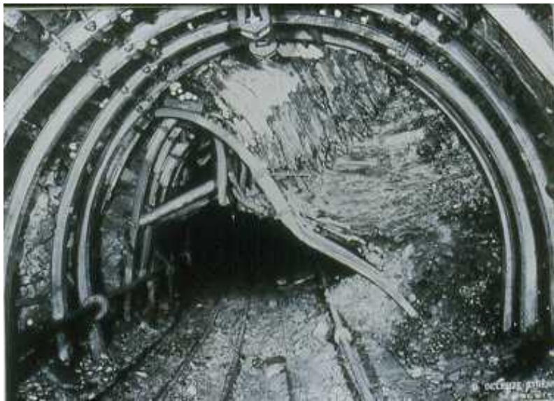
Ground failure in a Belgian coal mine, after a coal bump. The buckling of layers has been frozen in time and space by the steel support.
