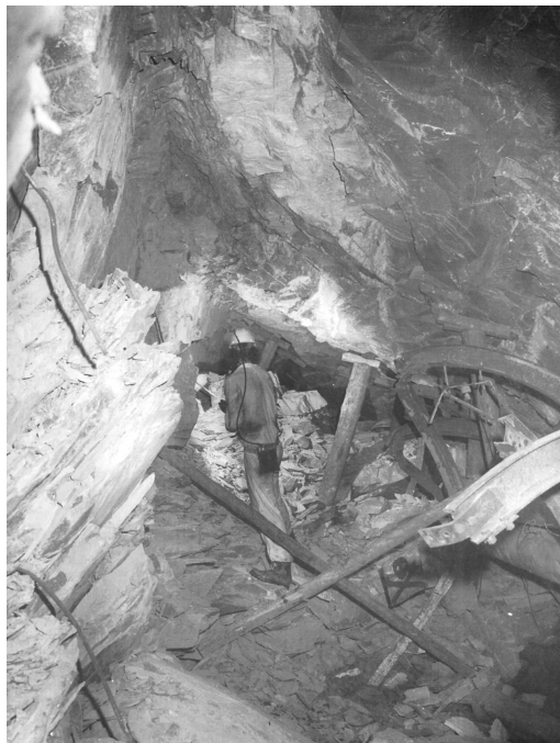
Asymmetrical roof failure in a South African gold mine under a rock burst (Courtesy of D. Ortlepp, 2003)
