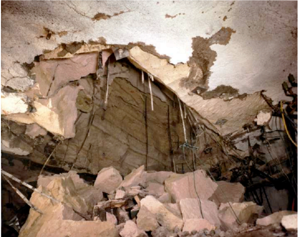
Fig. 39. Stable (?) roof arch created by a strong ground shock in volcanic tuff, Nevada, USA
