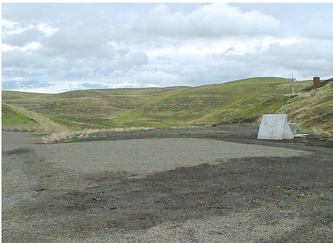
Figure 2. EWTF detonation pad.
