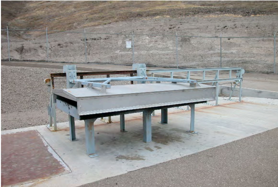
Figure 3. EWTF burn pan, covered. (UCRL-Photo-213179, July 16, 2005)
