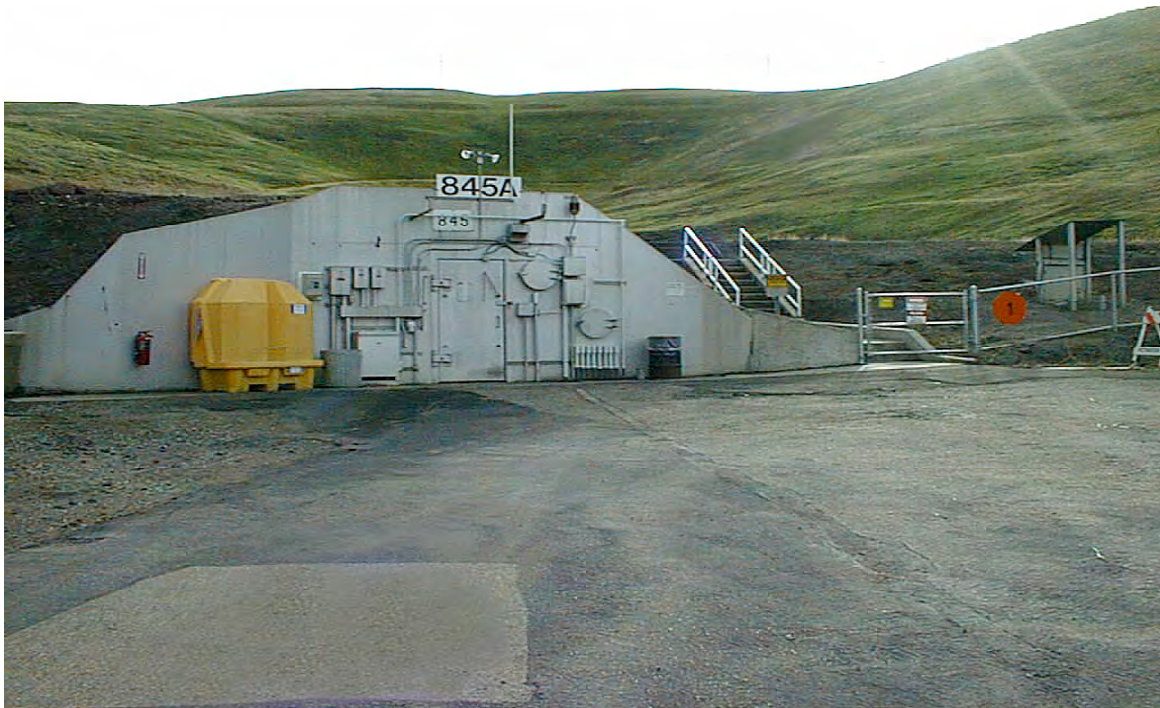
Figure 5. EWTF control bunker (Building 845A). Detonation pad is in the background.
