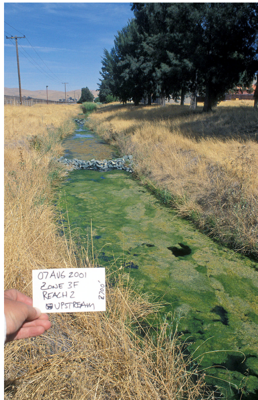
Figure 39. Photograph showing the lower end of Zone 3F (upstream view) with early succession annual and perennial grasses (upstream view). Open water habitat with significant algal growth was the dominant feature in 2001. Note rock weirs used for grade adjustment.
