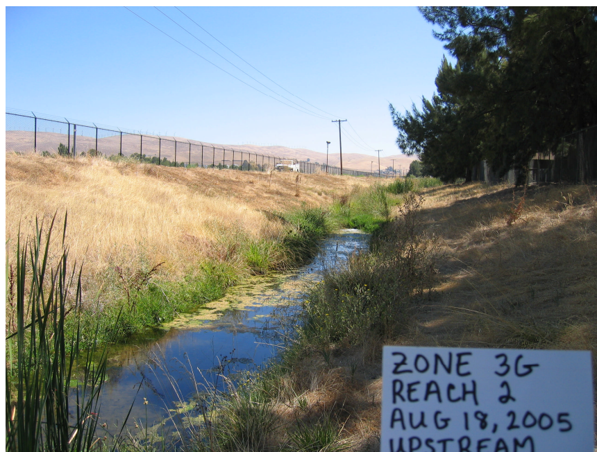
Figure 60. Photograph showing the lower end of Zone 3G (upstream view) five years after dredging with hydrophytes established.
