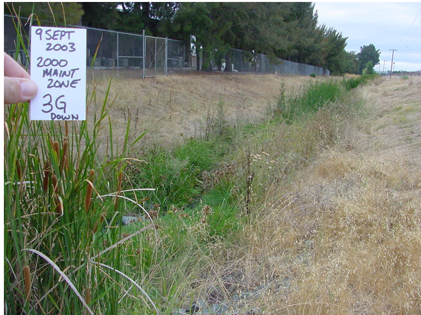
Figure 55. Photograph showing the upper end of Zone 3G (downstream view) three years after dredging with hydrophytes well established. Cattail establishment continued during this period.
