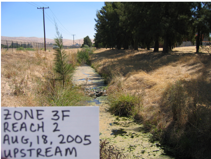
Figure 47. Photograph showing the lower portion of 3F (upstream view), essentially unchanged from previous years.
