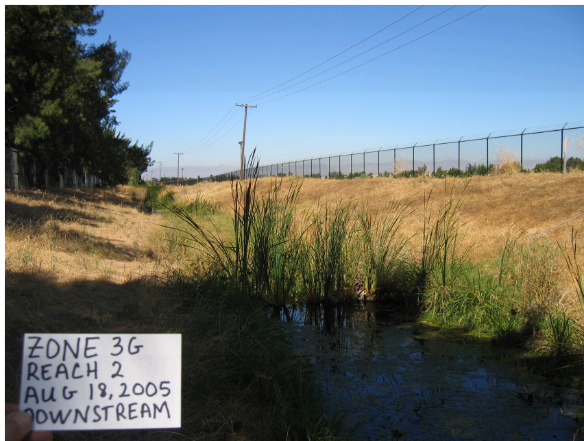
Figure 59. Photograph showing the upper end of Zone 3G (downstream view) five years after dredging with hydrophytes well established.
