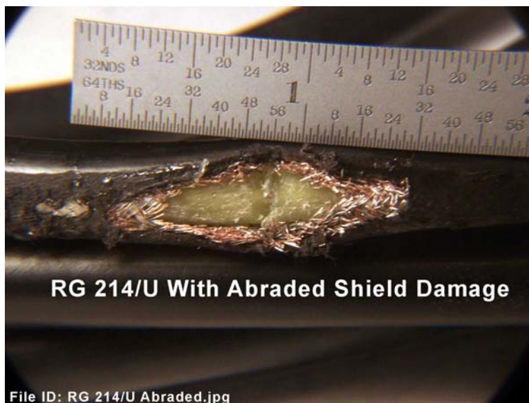
Figure 3: Abrasion on coaxial cable
