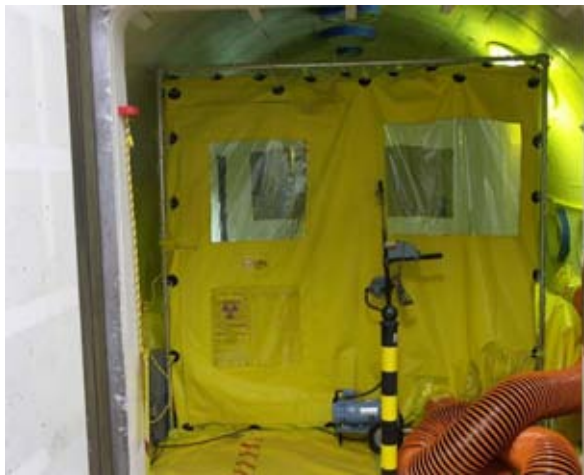
Figure 6.16 Phase 3 Secondary Enclosure Tent
