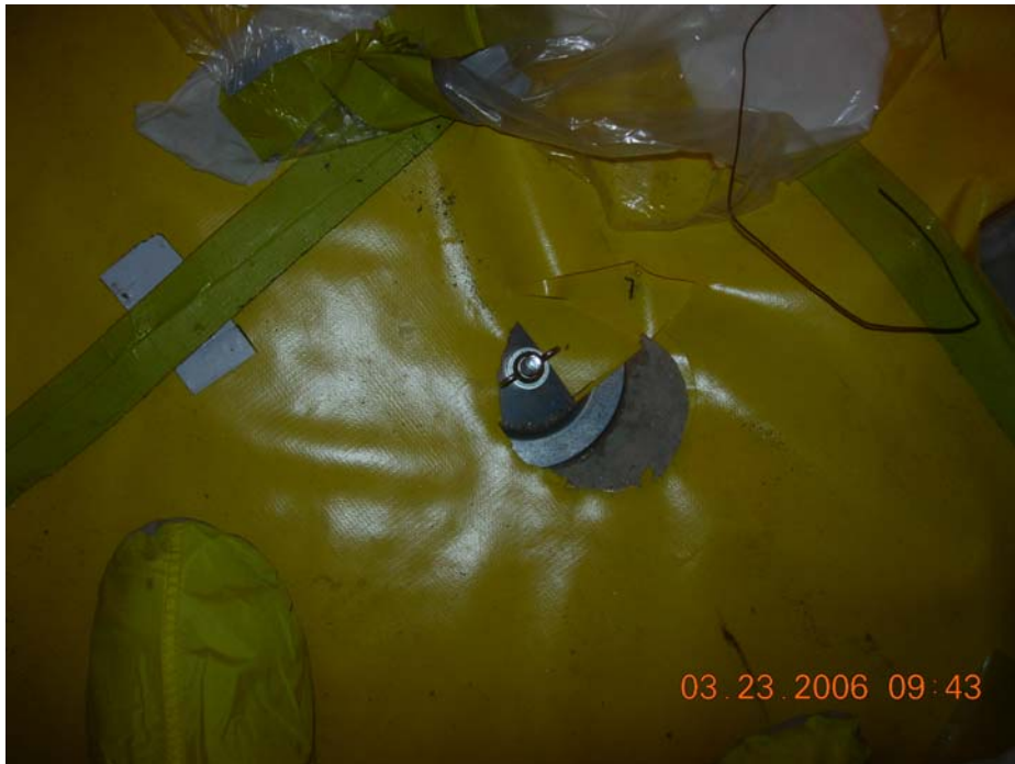
Figure 5. Isolation of the reactor drain tank containment vault floor drain.
