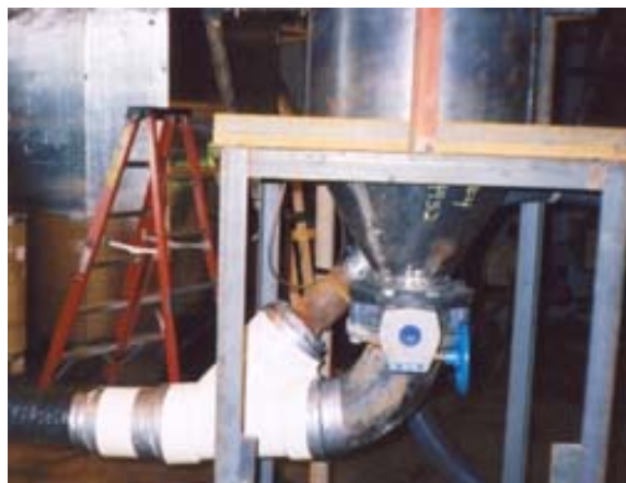
Photo No. 2. PFBR Discharge Section
