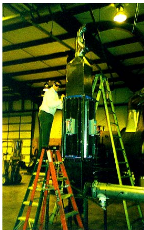
Photo No. 13. PFBR – Front View – Also Dr. Mazyck Conducting Inspection
