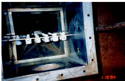
Photo No. 11. Rotatable Plenum Diffuser Plate - Open
