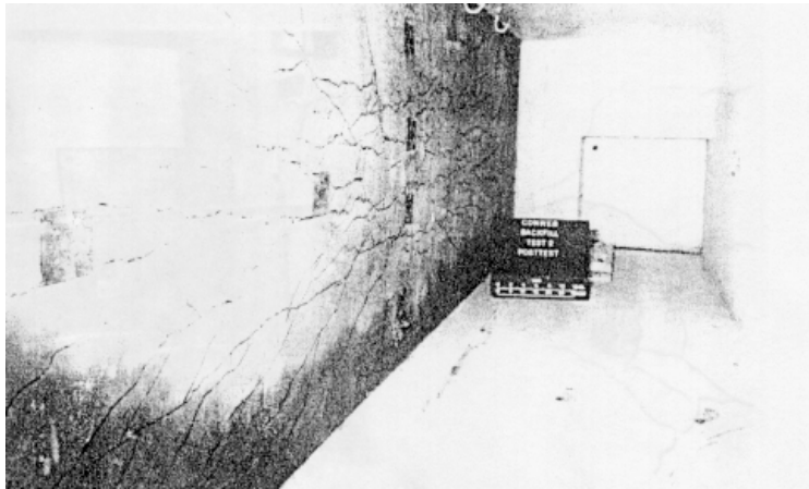
Figure 5-1. Interior View of RC Slab Damage (Courtesy of Hayes (1990))
