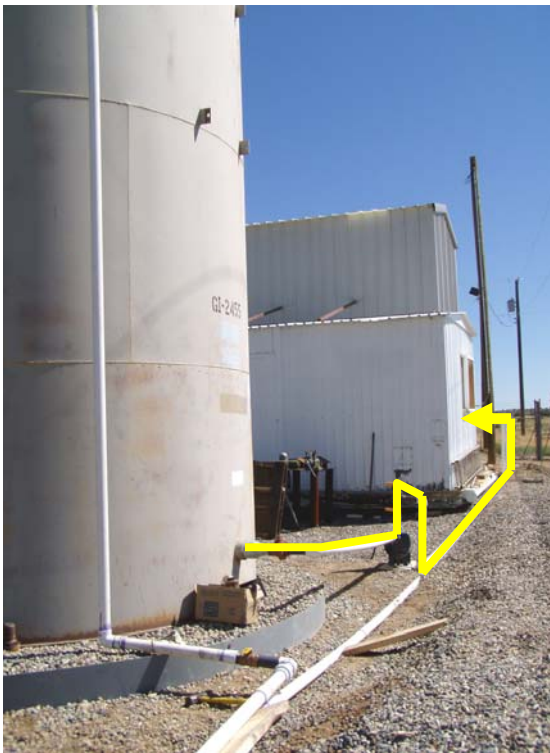
b) Produced water feed tank for SMZ columns
