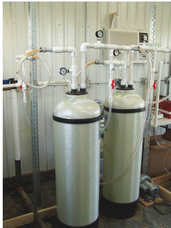
b) Produced water feed tank for SMZ columns
