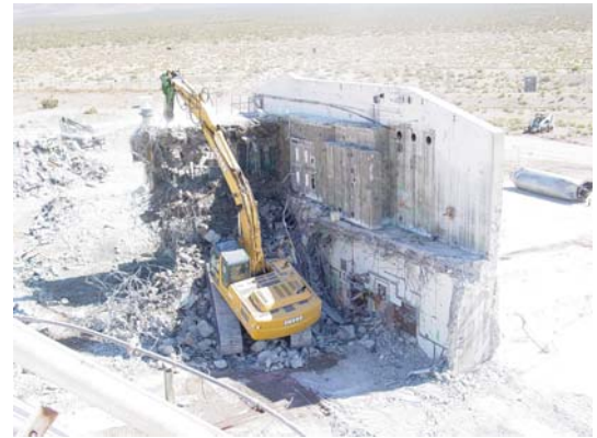
Figure 5. Mechanical Demolition
