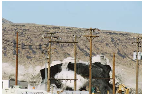
Figure 6. CED of Shield Wall
