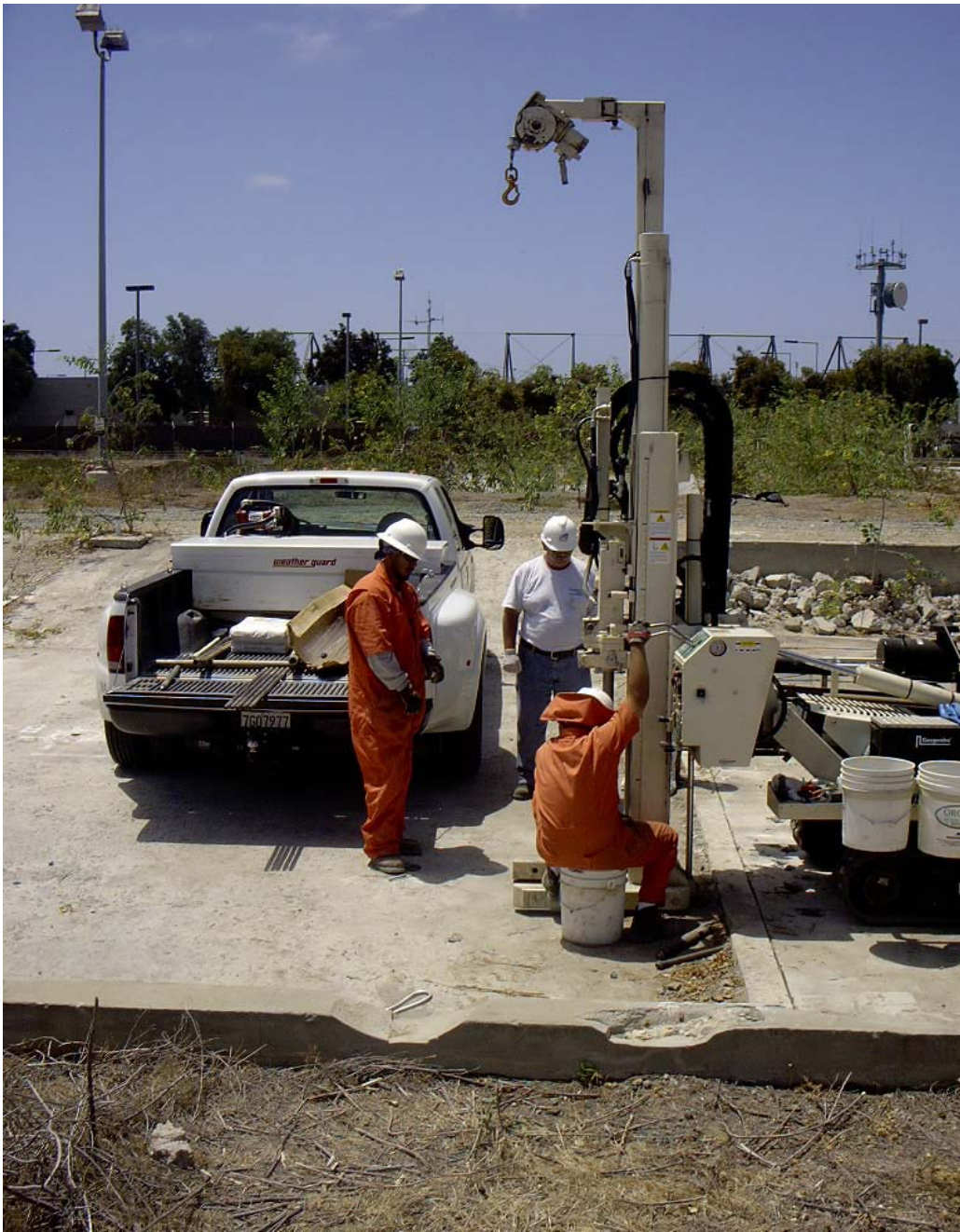
Figure 10. Geoprobe Equipment Being Used to Collect a Soil Boring for the Accu Core Validation Study
