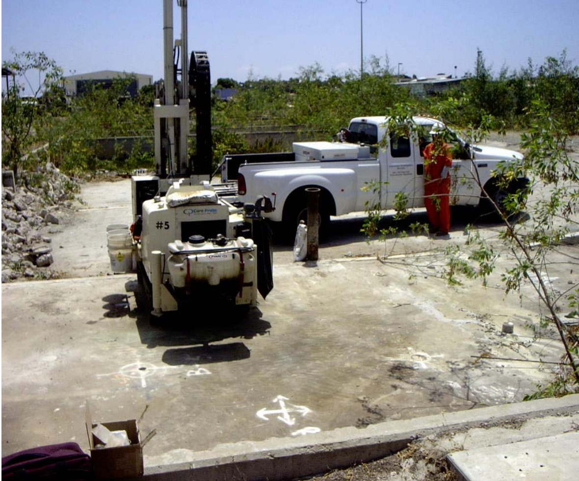
Figure 9. Geoprobe Equipment at the Accu Core Validation Study Sampling Site
