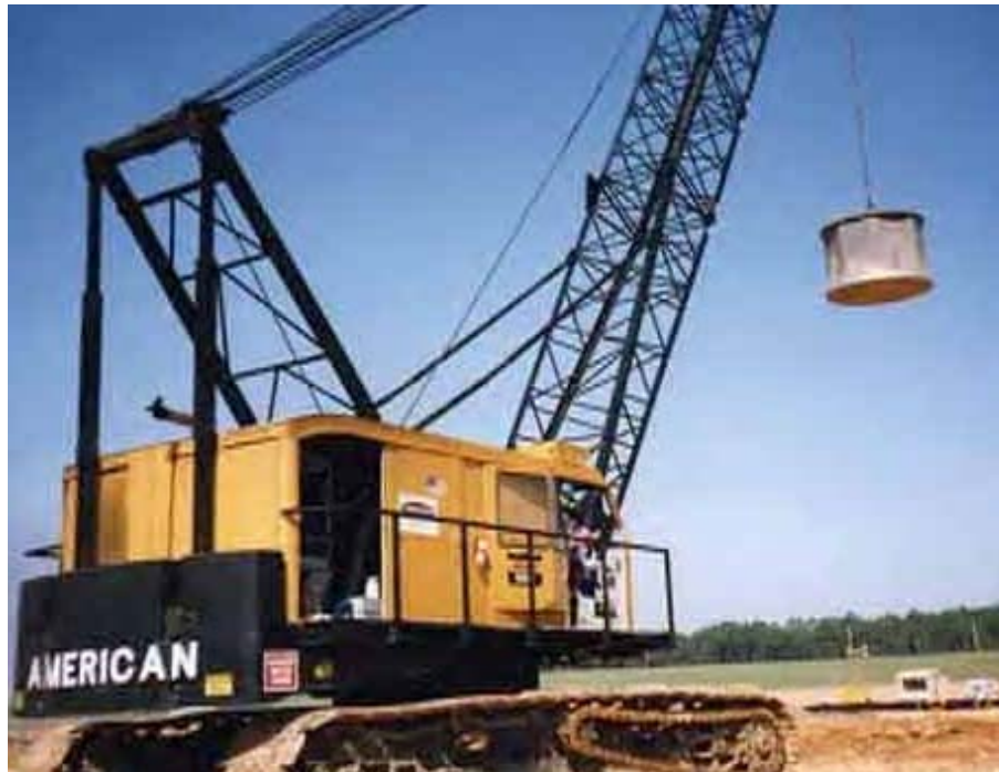
Figure E-25. Dynamic compaction operation at the Savannah River Site.
