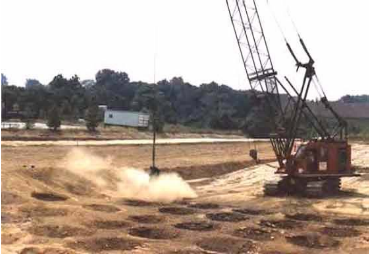
Figure 3-8. Dynamic compaction operation for Alternative 2b—Evapotranspiration Surface Barrier.
