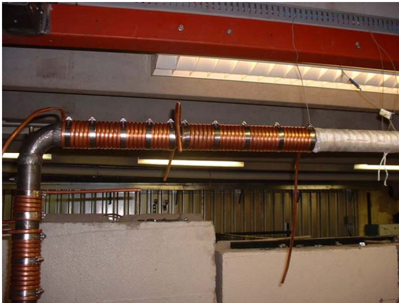
Figure 3-8 Cooling coils.
