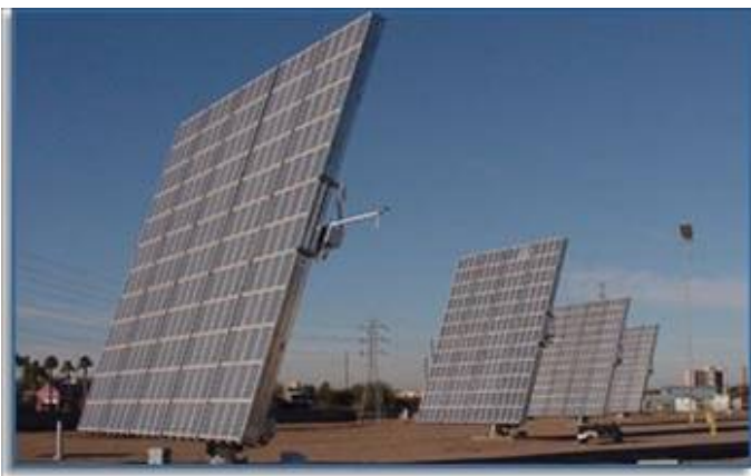
Figure 6-4. The 320-m 2 PV trackers at APS use hydraulic drives.
