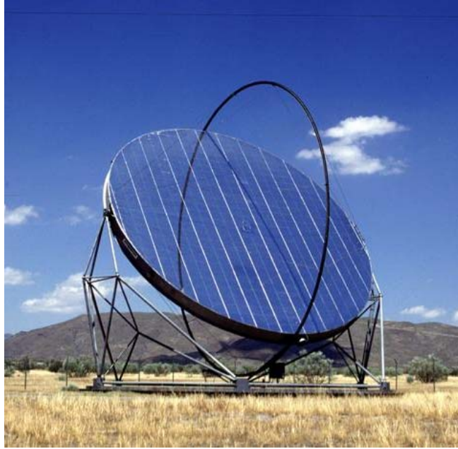
Figure 2-10. The ASM-150 heliostat built by SBP/Steinmüller.
