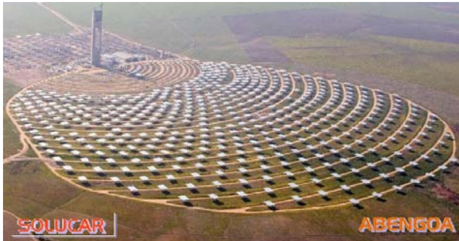
Figure 2-7. In 2006, PS-10 (near Seville, Spain) uses 624 pedestal-mounted heliostats built by Solucar. Each heliostat is 121 \text{ m}^2 for a total area of 75,504 \text{ m}^2 .
