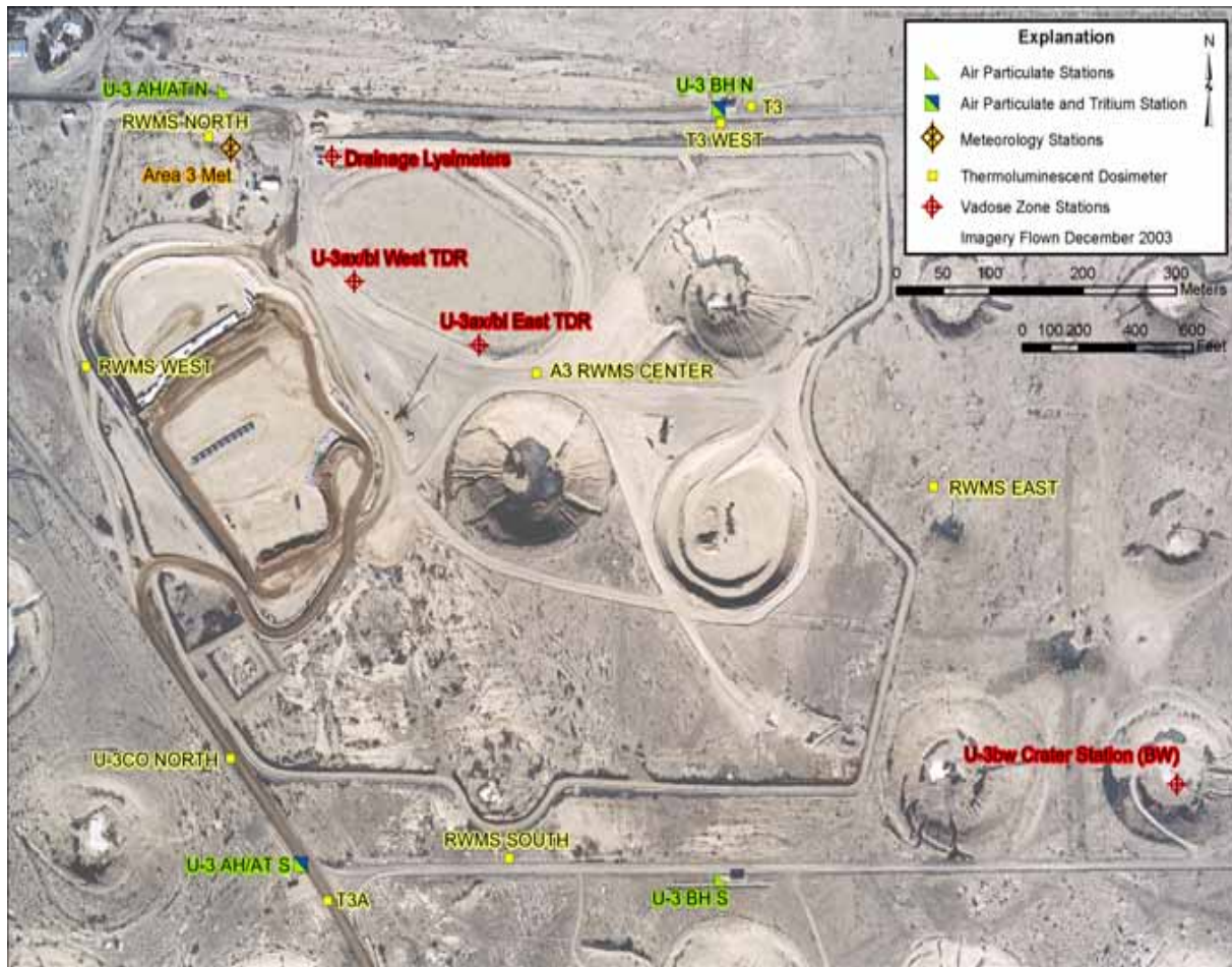
Figure 5 Monitoring Stations at the Area 3 RWMS
