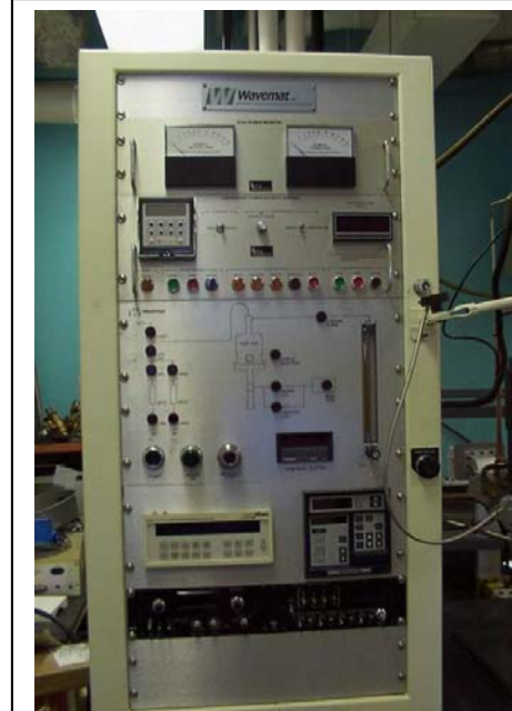
Figure 3.3 Control panel of microwave power (Microwave power is adjustable)
